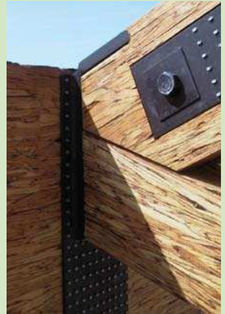
Conventional column and beam hardware can be used with Parallam® PSL beams.
