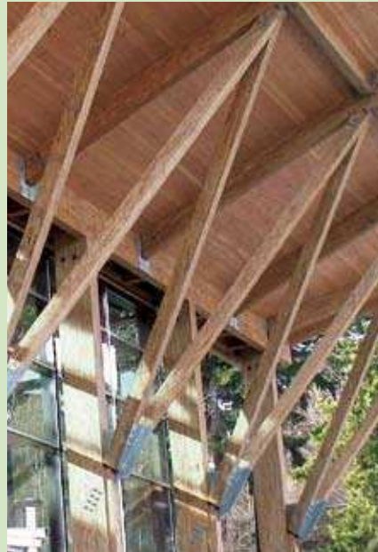
Parallam® PSL columns and beams combine to form an exceptionally strong and rigid framework.
