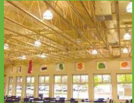
This school cafe uses open-web trusses to easily and efficiently create large open areas.
