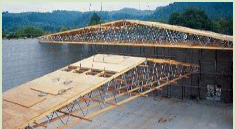
TJH™ trusses—60 feet long and up to 6 feet deep—form the structural backbone of this 12-acre reservoir cover, which was specially engineered to withstand both vertical and horizontal loads.
