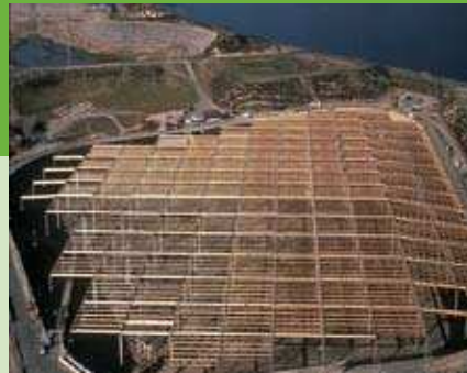
TJH™ trusses—60 feet long and up to 6 feet deep—form the structural backbone of this 12-acre reservoir cover, which was specially engineered to withstand both vertical and horizontal loads.
