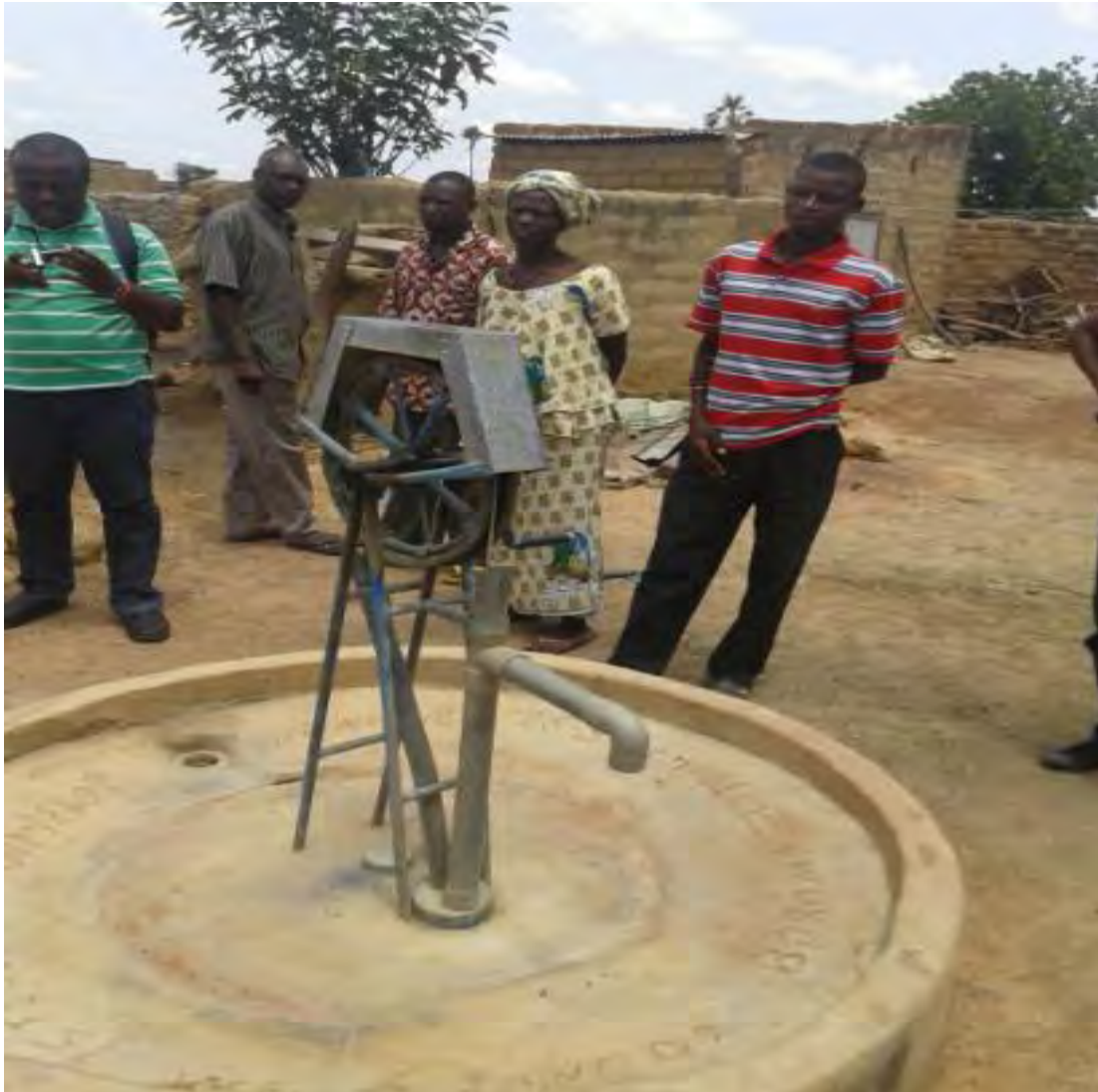
Figure AN 5: A rehabilitated well at Oullo in Burkina Faso
