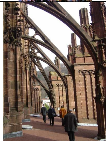
Flying Buttresses on the Bourges Cathedral (built 1195-1230)
