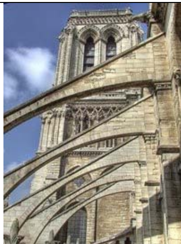
Flying Buttresses at Notre Dame Cathedral, giving masonry support to the walls of the nave.
