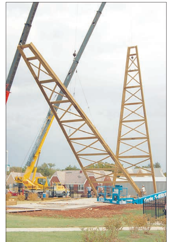
Raising the derrick legs (Everett photo).
