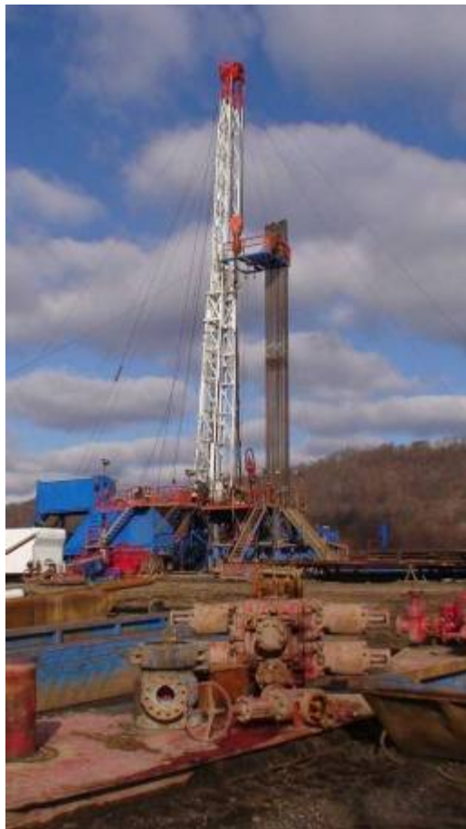
Drill rig on site (Jan 2007)
