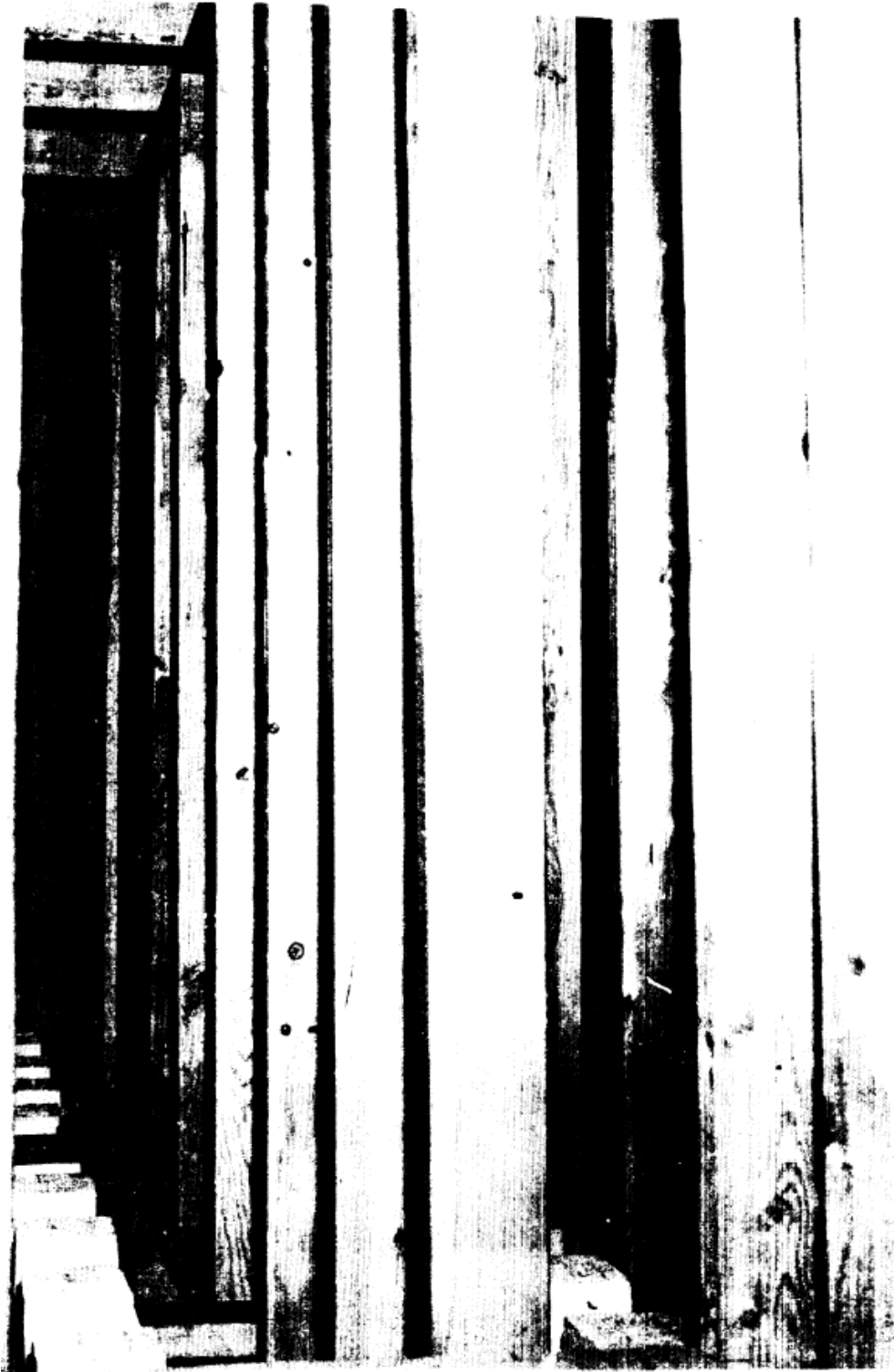
Figure 42: View along left side of furnace blocking
