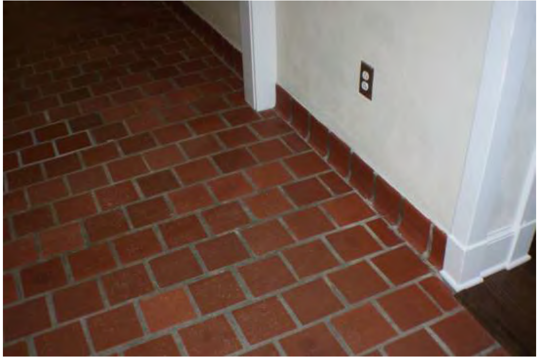
Cleaned quarry tile floors at Ohio Hall
