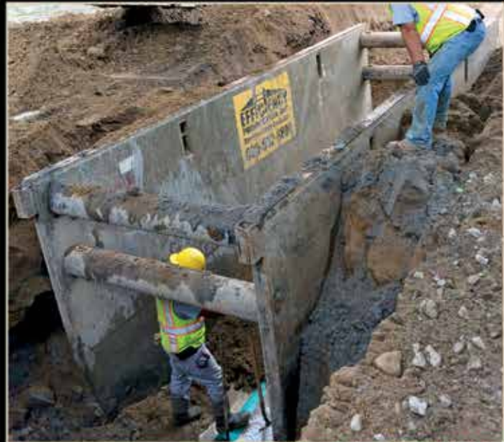
Steel Trench Shields
