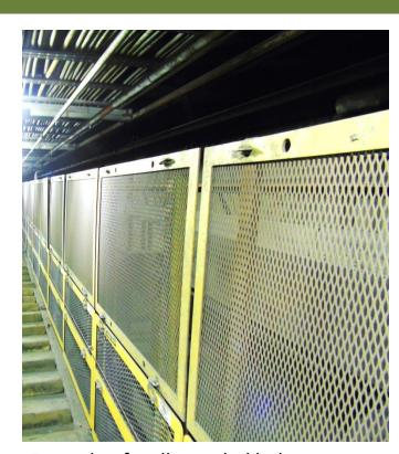
Example of well guarded belt conveyor pinch points and rotating parts; movable guards are equipped with wedge clamps.
