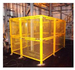
Single conveyor gravity take-up counterweight guarding (source: Belt Conveyor Guarding)
