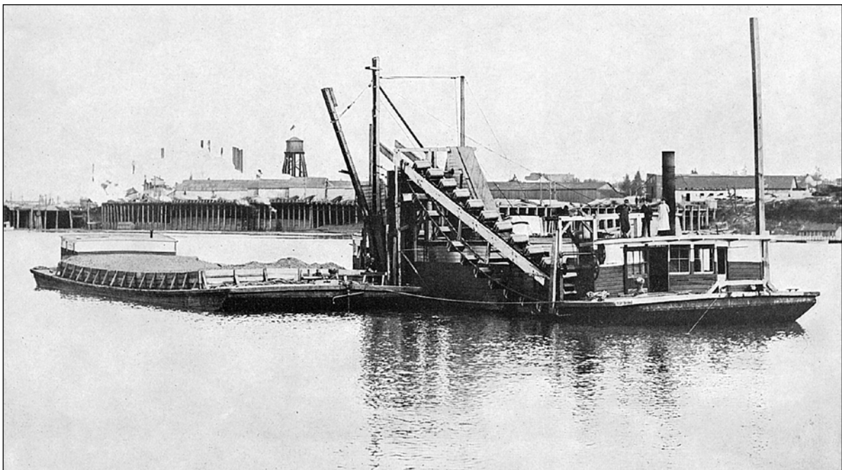
Figure 3.10: Dredge for raising sand and gravel from the bed of the Willamette River near Portland, Oregon, Circa 1909 (Langer, 2003)
