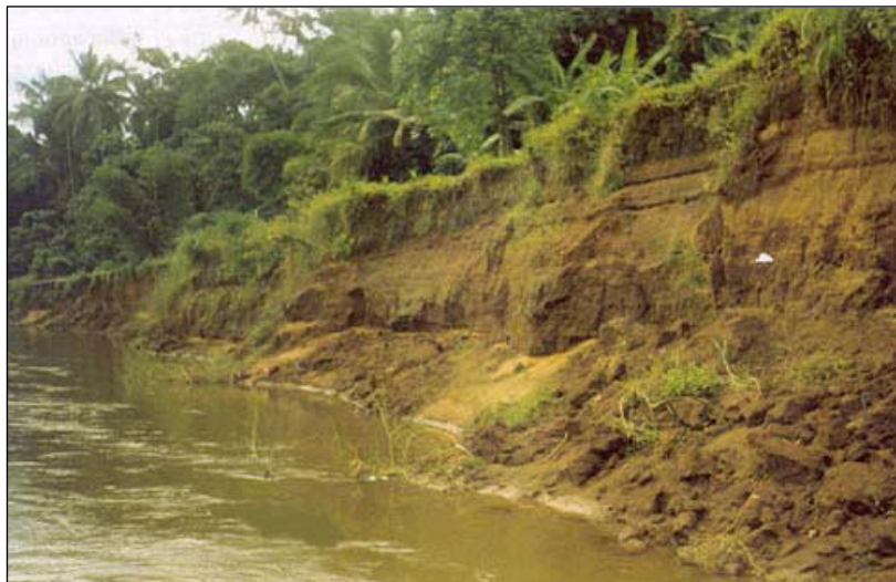
Figure 2.12: Slumped/Exposed Bank of Pamba River Due to Unrestricted Mining Activities (Padmalal et al., 2008)
