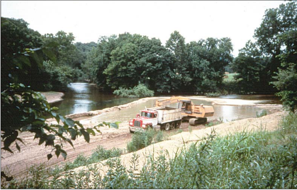
Figure 3.8: Aggregate being “skimmed” off the surface of a bar (Langer, 2003)
