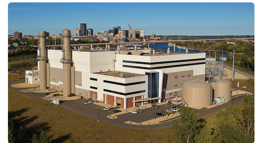
Converted for natural gas production, the Xcel Energy High Bridge Generating System in Saint Paul came on line in May 2008.
