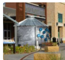
Maplewood Mall 55 rain gardens, 6,733 square feet of permeable pavers, 375 trees, and one decorative 5,700-gallon cistern built to catch stormwater greet visitors. Together, they help intercept 20 million gallons of runoff per year before it reaches nearby Kohlman Lake.
