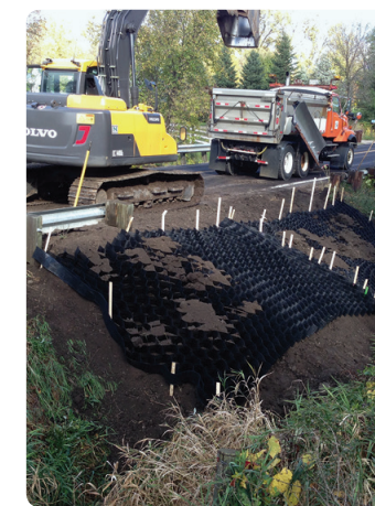
Flooding in 2012 in Northeast Minnesota damaged roads and bridges, water and sewer systems and other infrastructure, costing $108 million. More than 1,700 homes and 100 businesses were damaged or destroyed, costing more than $12 million.
