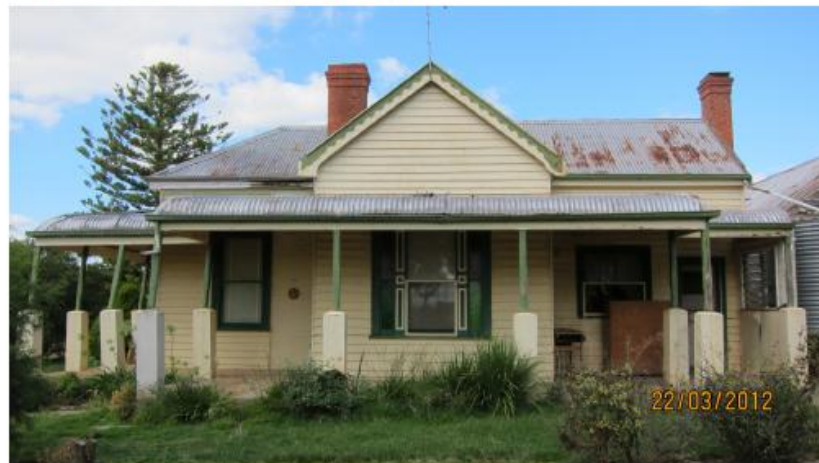
Farmhouse dating from c 1900. The verandah pillars are an alteration.
