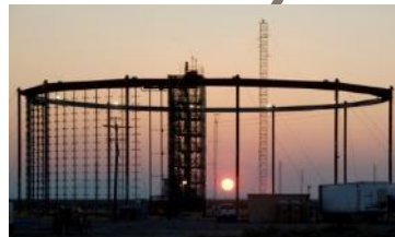
Infrastructure in place with state-of-the-art equipment
