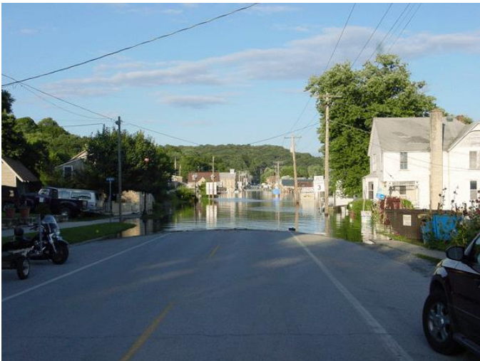
Flooding along The Great River Road (Highway 100) near the intersection of Highway 3 (looking east)
