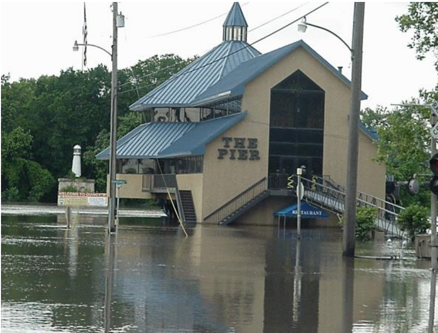
Flooding of The Pier Restaurant in Quincy, Illinois
