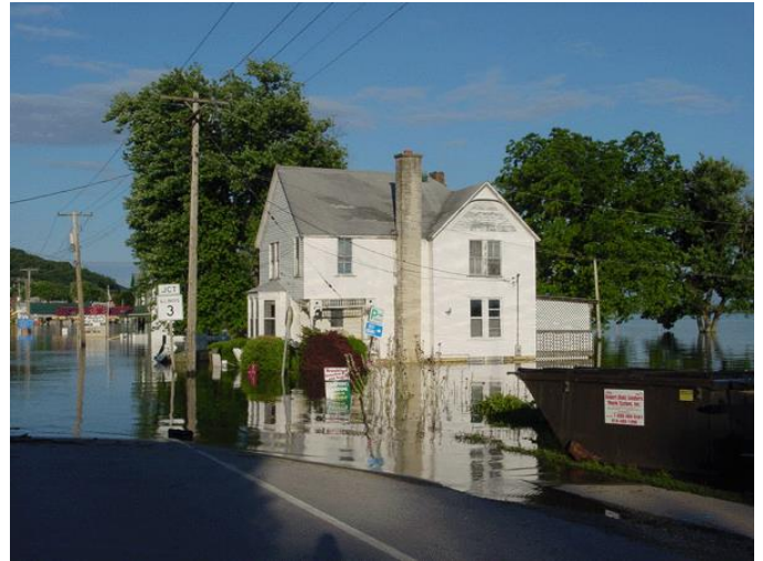
Flooding along The Great River Road (Highway 100) near the intersection of Highway 3 (looking east)
