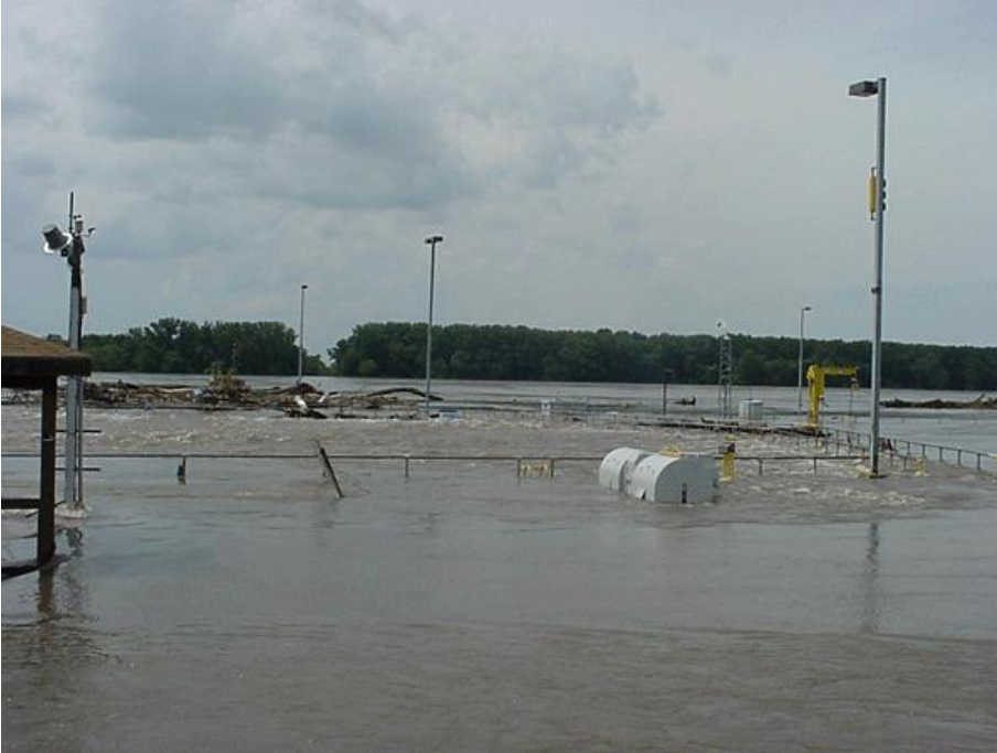
Flooding of Quincy Lock and Dam 21
