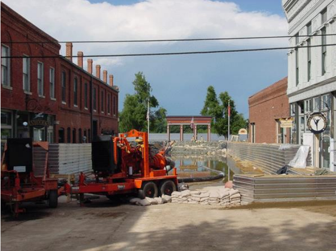
Flood Control on Howard Street in Clarksville
