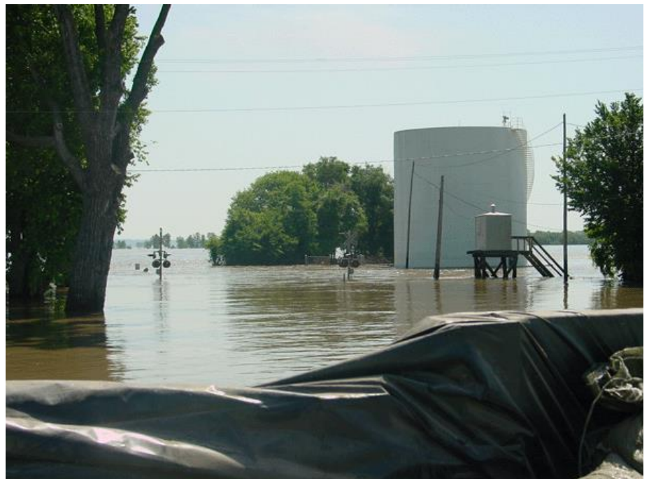
Flooding north of downtown Canton, Missouri
