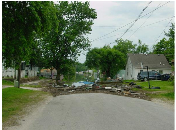
Flooding and debris covered the streets of Louisiana, Missouri
