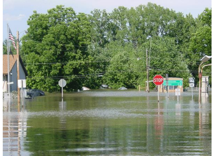
Flooding along Highway 79 in Clarksville
