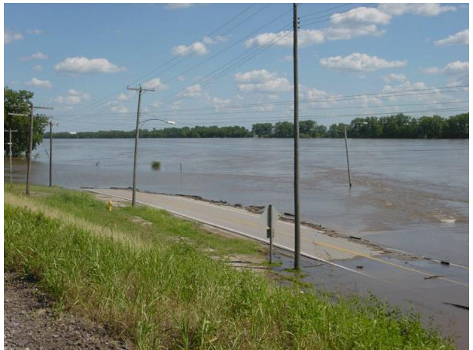
Flooding of Water Street in Chester, Illinois
