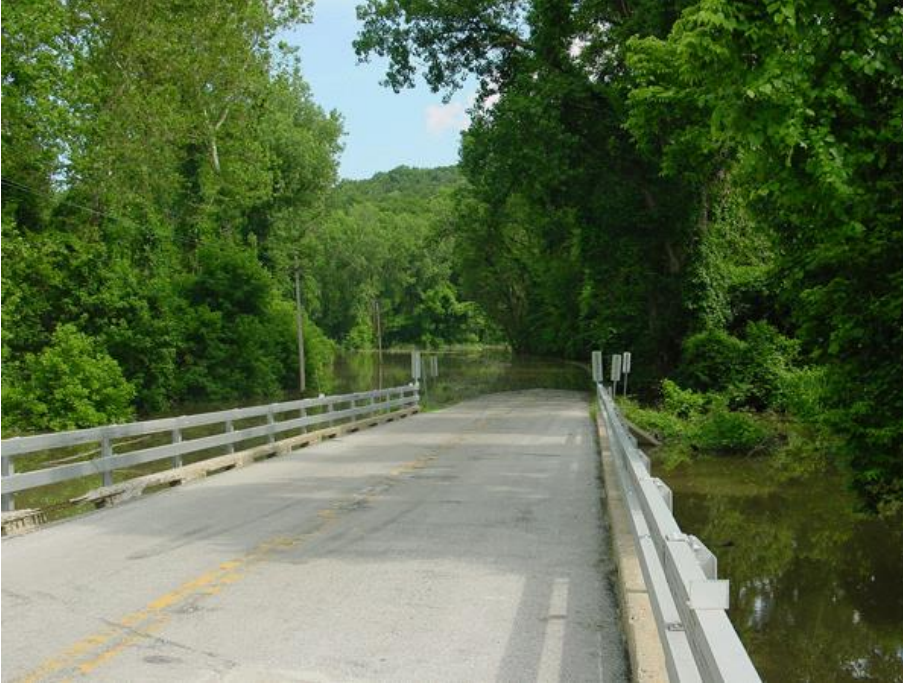
Flooding of Highway E near Saverton, Missouri
