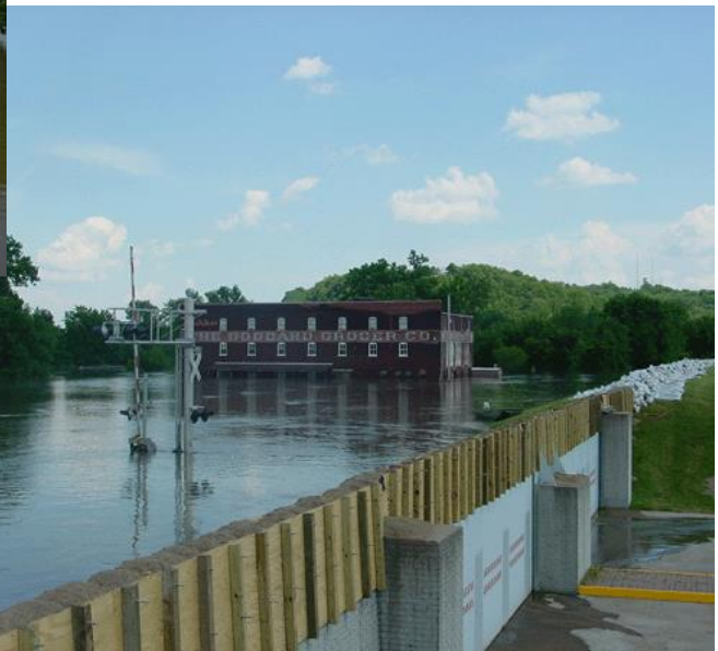
Broadway Street Flood Wall in Hannibal, Missouri (looking southeast)
