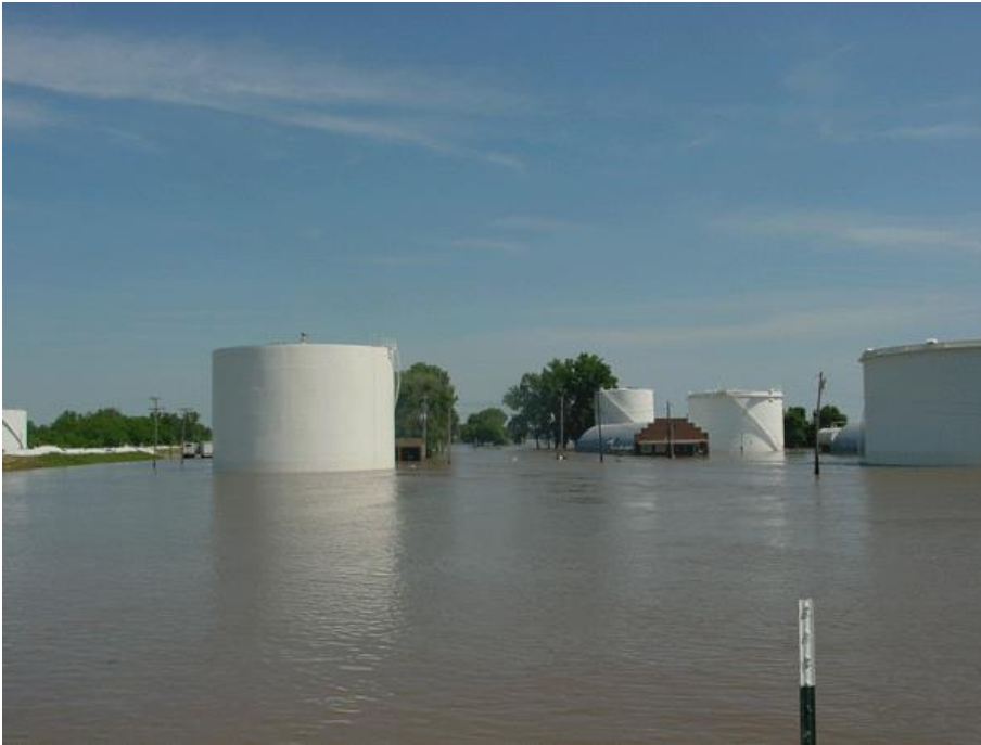
Flooding near Grant Street in Canton, Missouri
