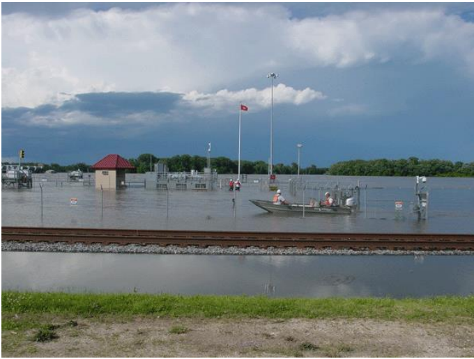
Flooding of the Clarksville Lock and Dam
