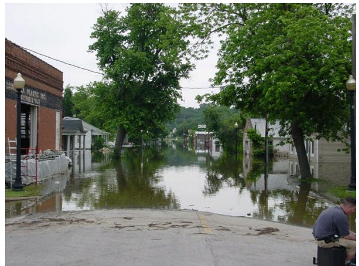
Flooding of Highway 79 in Louisiana, Missouri
