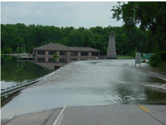
Flooding along Highway 54 Bridge near Louisiana, Missouri (looking east)
