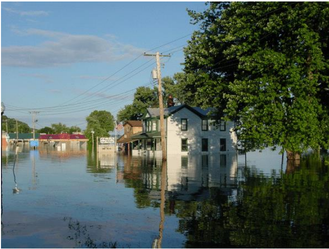
Flooding along The Great River Road (Highway 100) in Grafton, Illinois
