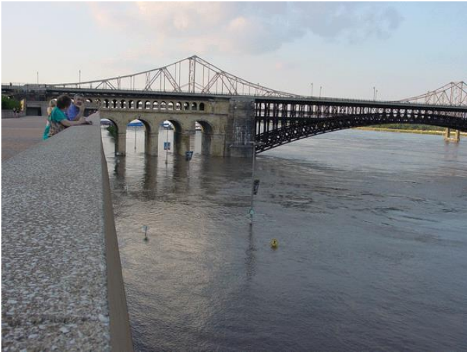
Mississippi River flooding near the Eads Bridge (looking north from the flood wall)
