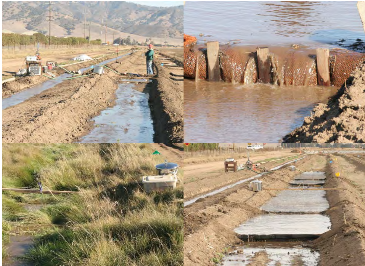
Figure 1. Examples of the Year 1 treatments on the USDA Spence Road farm. Clockwise from top left: bare ditch, compost sleeve, granulated activated carbon sleeves, and vegetated ditch.
