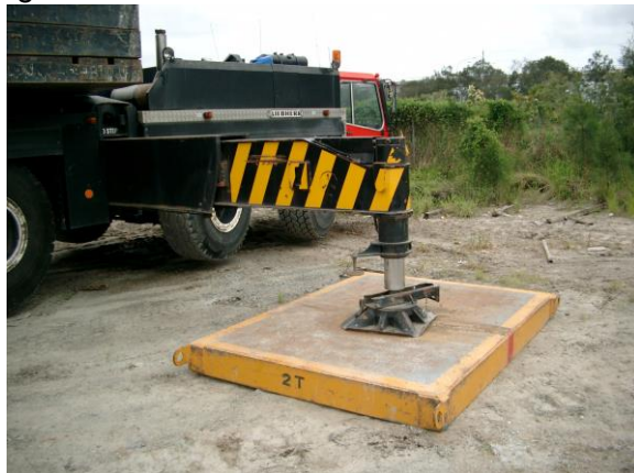
Figure 4 - Crane outrigger foot on bog mat
