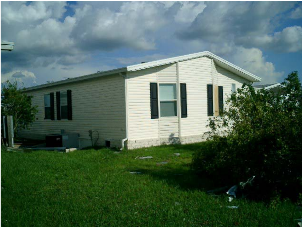
Figure 6.18: Manufactured Home Survived the Hurricane Wind Forces
