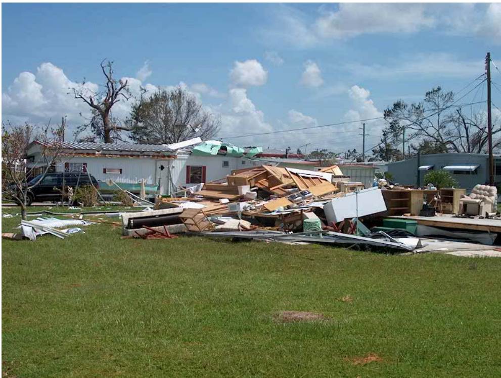
Figure 6.8: Destroyed Manufactured Home Built Prior to 1976
