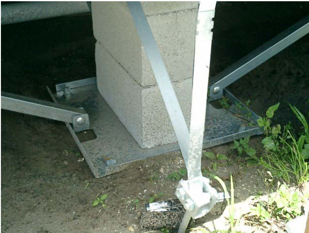
Figure 6.38: Scouring Action of Wind and Rain Water Runoff
