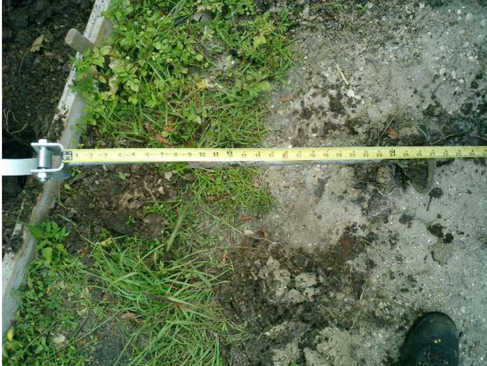
Figure 6.25: Manufactured Home Installed with Short Ground Anchors
