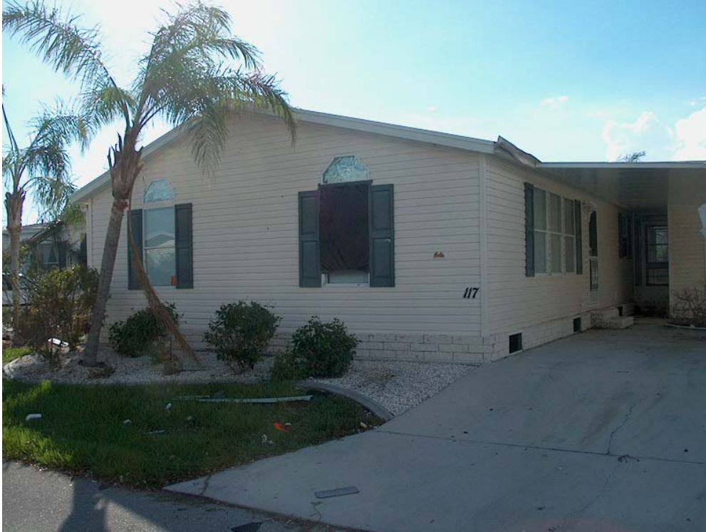
Figure 6.19: Manufactured Home Survived the Hurricane Wind Forces
