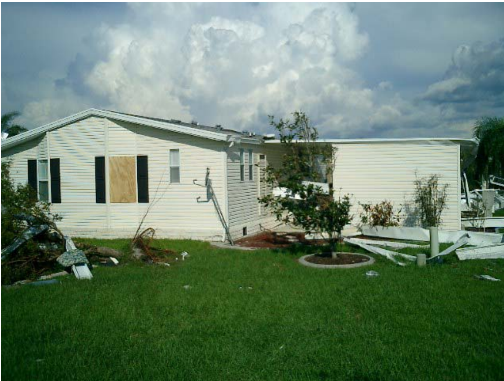
Figure 6.20: Manufactured Home Survived the Hurricane Wind Forces
