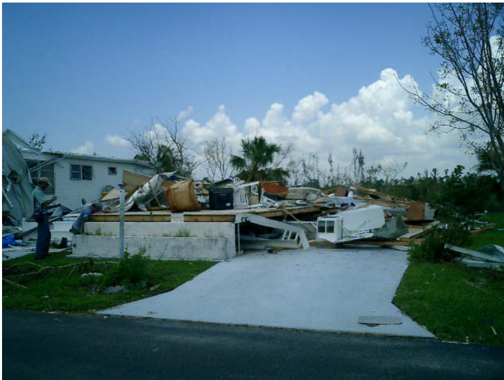
Figure 6.16: Destroyed Manufactured Home
