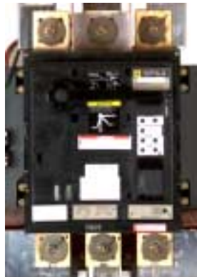
Thermal Magnetic Circuit Breaker
