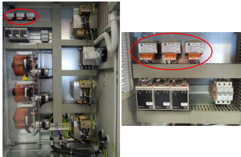
Fig. 11. Three single-phase Measurement Transformers
