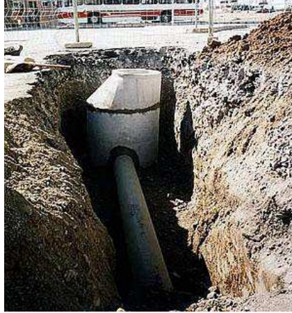
Figure 8. Construction of a manhole and connection to the sewer pipe
