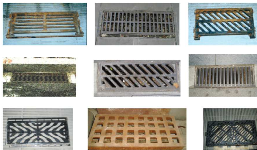
Figure 7. Different grate models. Taken from Gómez and Russo, 2010
