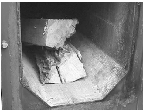
Correct way to load wood. Use 2-3 hardwood logs, 4-6 inches in diameter, 12-15 inches long.
