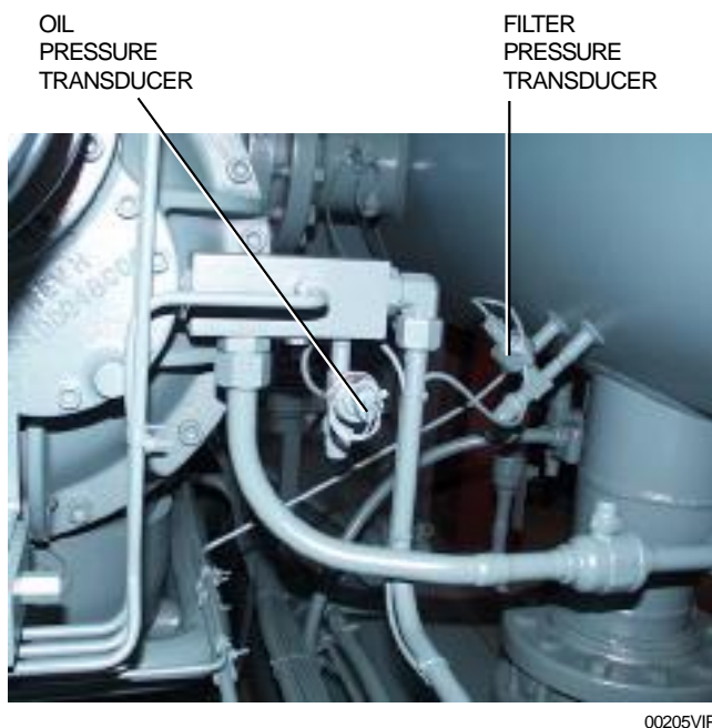
FIG. 18 – OIL AND FILTER PRESSURE TRANSDUCERS
