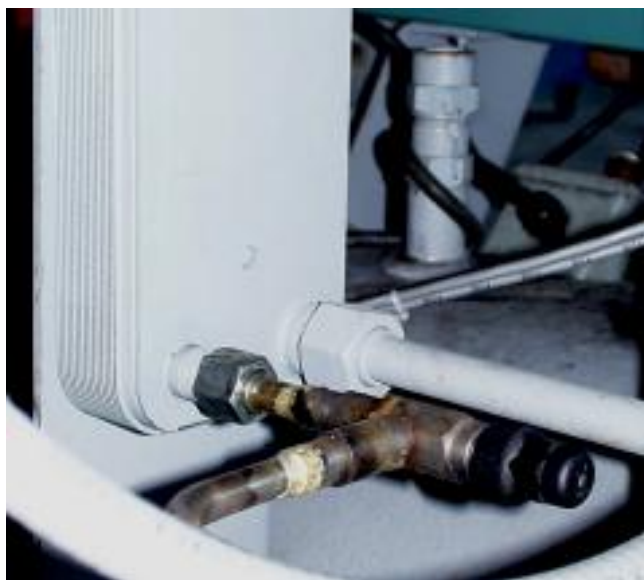
FIG. 29 – OIL COOLER VALVE
