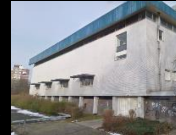
KPN telephone exchange: detector location
