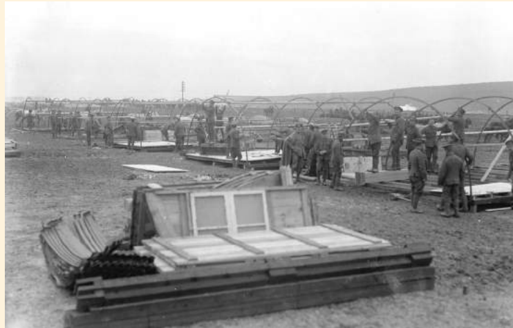
British troops constructing Nissen huts, Fricourt, 1916
