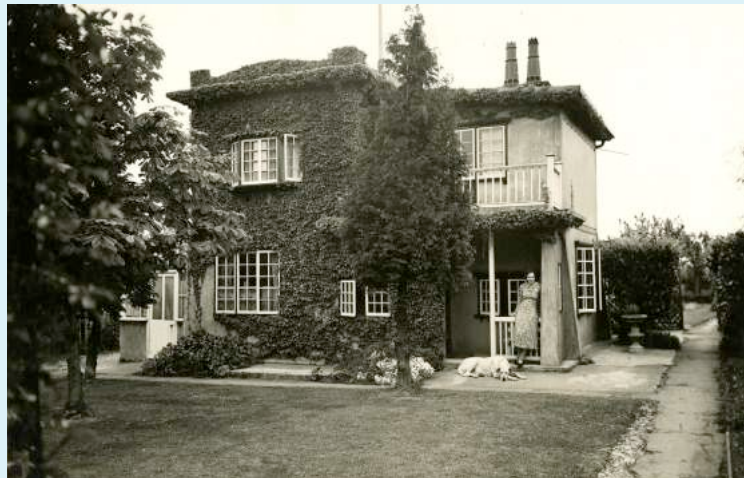
158 Wilbury Road, Letchworth, 1905, Grade II* listed both for its style and its radical prefabricated reinforced concrete construction
