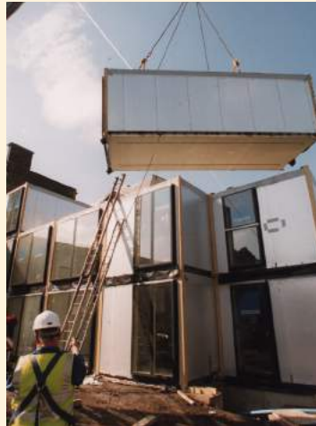
Murray Grove, London, pioneered steel framed volumetric construction in 1999
