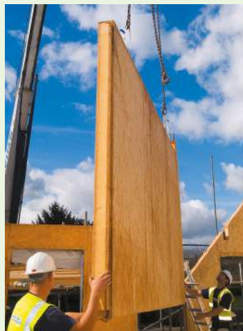
SIPS (structural insulated panel systems) Kingspan TEK building system
