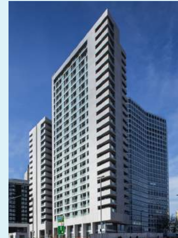
Arena Central, Birmingham, 2019 using up-to-date precast construction
