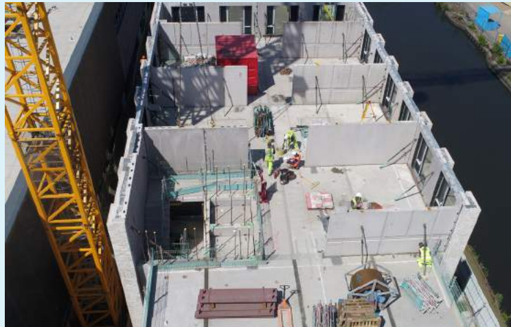
Example of precast concrete cross wall construction, a fast and convenient way to produce multi-unit structures
