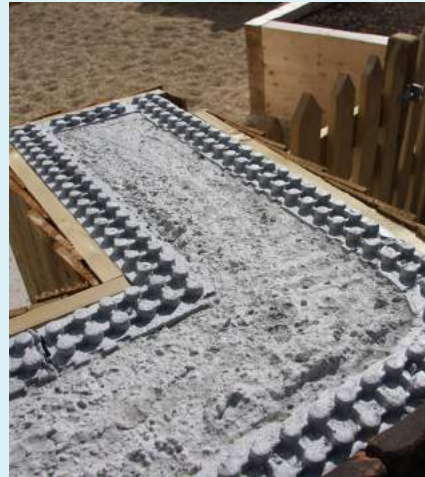
Concrete is poured into the insulating formwork at Chewton Mendip cottages
