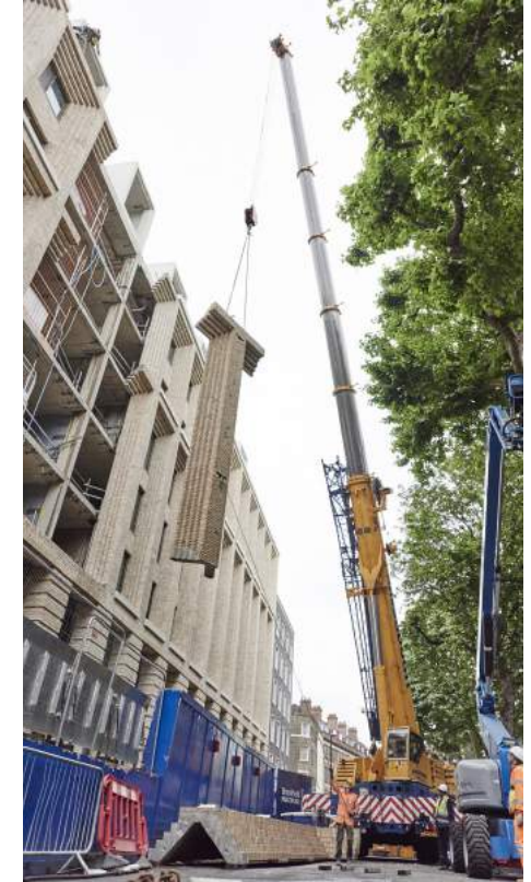
Garden Halls student accommodation, London, 2017, brick-faced precast concrete façade
