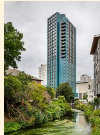
Mapleton Crescent: insulation, cladding and façade applied onsite
