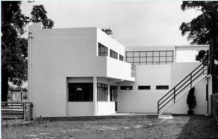
Class E House, Modern Homes Exhibition, 64 Heath Drive, Gidea Park, London, view of the house from the south-west showing the terrace
