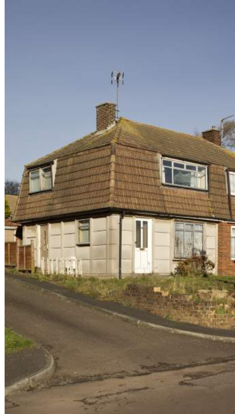
Cornish Unit precast houses at Hoo Peninsula, Medway, Kent. Thirty thousand built 1946–1960s
