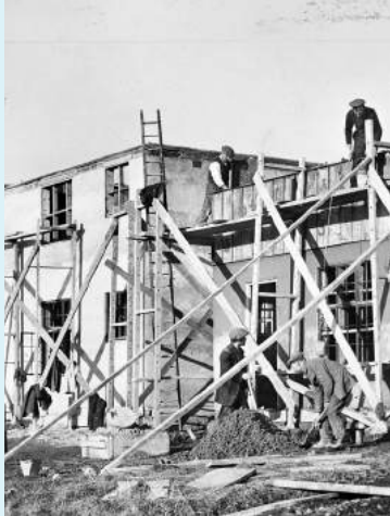
Easiform cast-in-situ concrete housing being constructed in 1926
