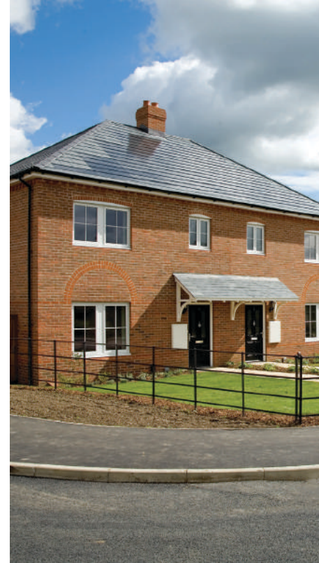
Brookwood Farm, Woking, 2009 insulating concrete formwork construction traditional looking houses
