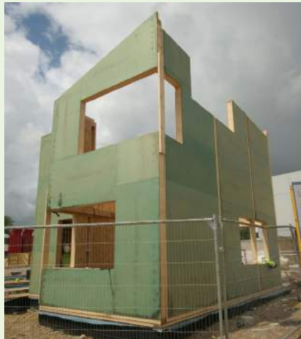
Oxley Woods panellised timber frame: complete wall panels and floor cassettes
