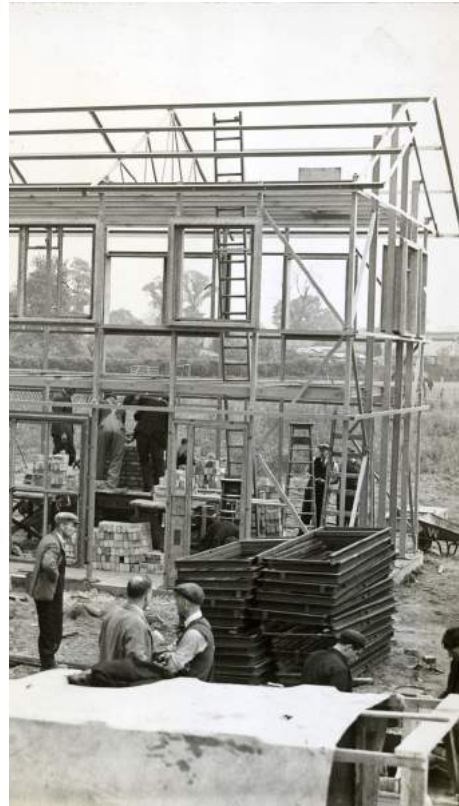
BISF prefabricated house at Ministry of Works' testing ground, Northolt, London, 1939–1945
