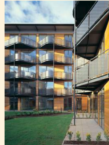
Murray Grove level access over thresholds on the garden side
