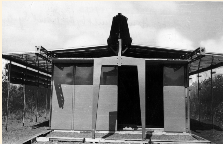
Maison Tropicale by Jean Prouvé under construction, 1951
