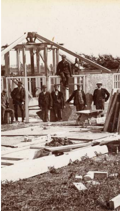
Cubitt's reinforced concrete 'The Roundhouse', Cheap Cottages Exhibition, Letchworth, 1905
