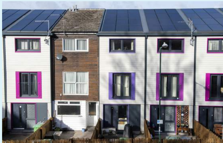
NCH 2050, the UK's first Energiesprong renovation pilot completed in 2018
