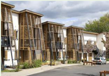
Hanham Hall deep roof overhangs, balconies and shutters help avoid overheating in summer
