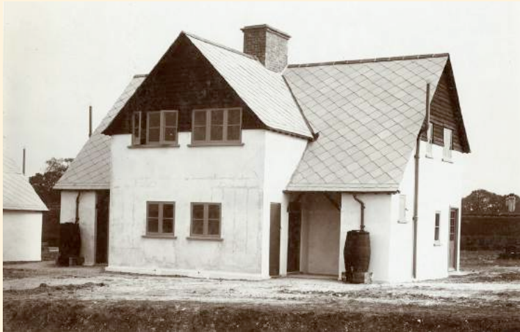
Letchworth Cottage No. 47 by New Expanded Metal Co. Ltd, 1905. Innovative use of metal lathing as a base for external render and internal plaster finish
