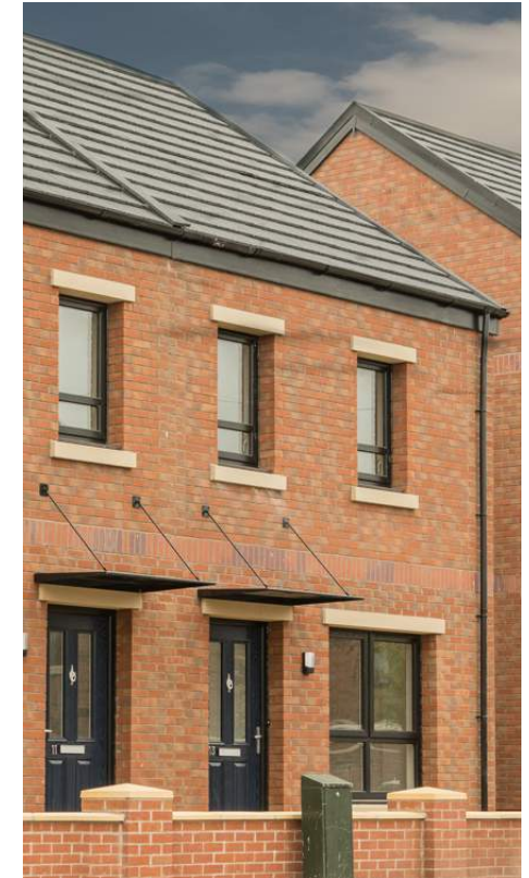
St Hilda's, Leeds, 2018, panellised construction using light steel frame for low-rise family homes
