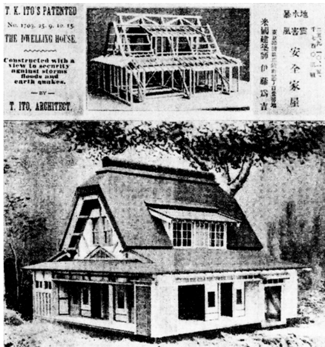
Figure 10: A seismic proof house proposed by Tamekichi Ito soon after the earthquake in 1891 (source: S. Matsumura, Jutaku ga dekiru sekai no shikumi, Shoukoku-sha, Tokyo, 1998).
