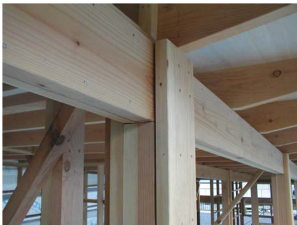
Figure 17 and 18: Structural details, House in nailed planks post-beam.
