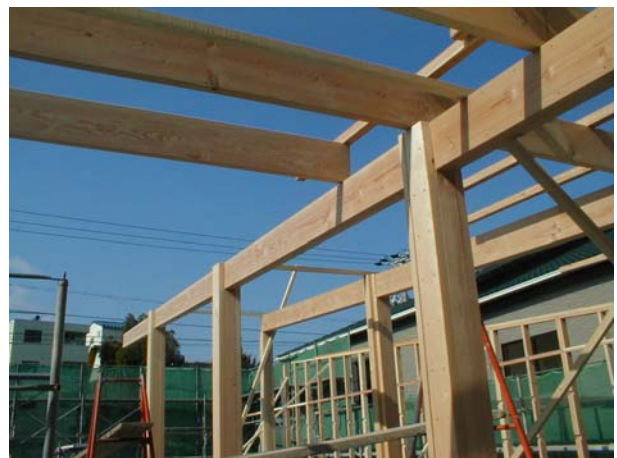
Figure 17 and 18: Structural details, House in nailed planks post-beam.
