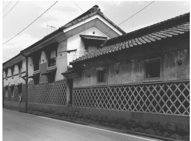
Figure 9: Warehouse with "Namako-kabe wall" (photo: Yasunao Hayashi).
