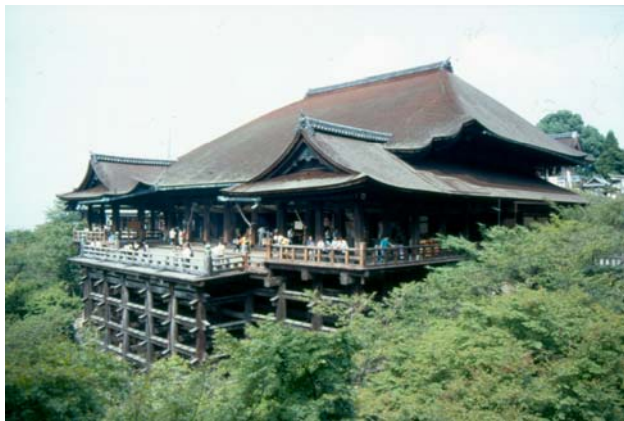
Figure 1: Kiyomizu-dera built on timber pilotis, early 17th century in Kyoto (photo: Wolfgang Winter).
