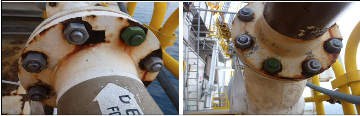
Figure 1. Typical Field Trial Installation
