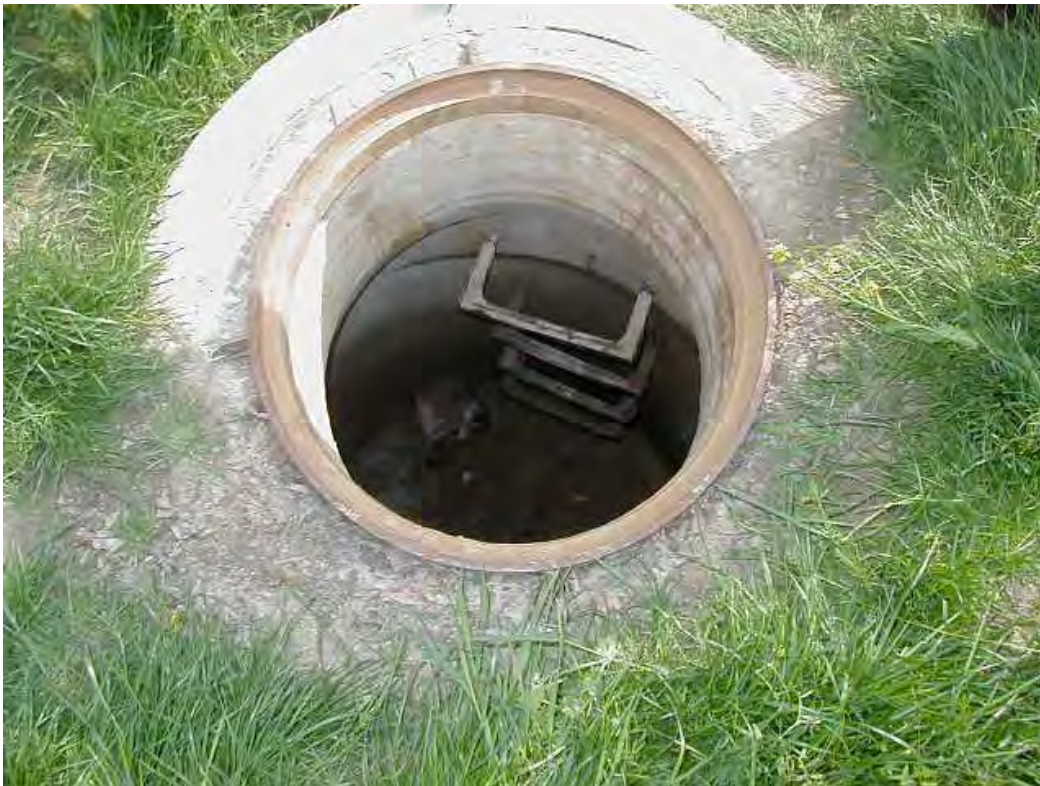
Figure 1. The landfill manhole where the fatality occurred.
