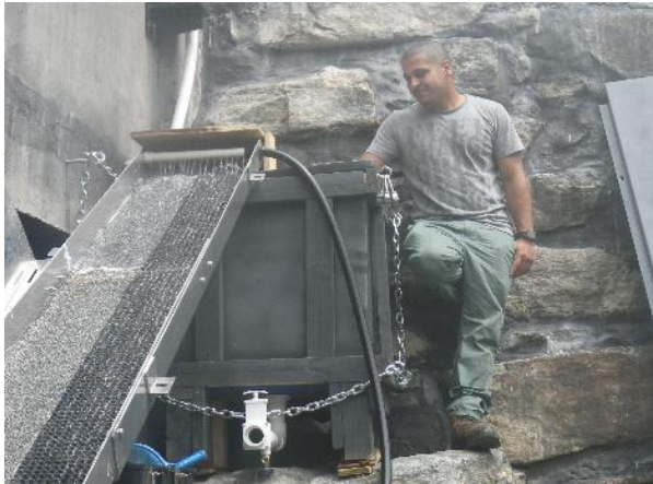
Photo 22: Location to stand adjacent to the holding tank
