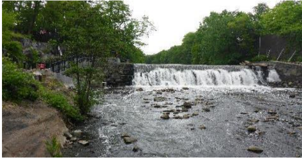
Photo 2: Looking upstream at the East 182 nd Street Dam
