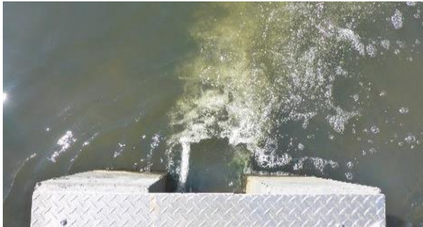
Photo 5: Fish entrance to the fish ladder
