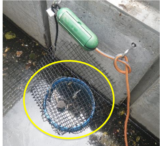
Photo 29: Water pump (inside yellow circle) that supplies water to the eel passage; located inside the fish ladder near the exitway
