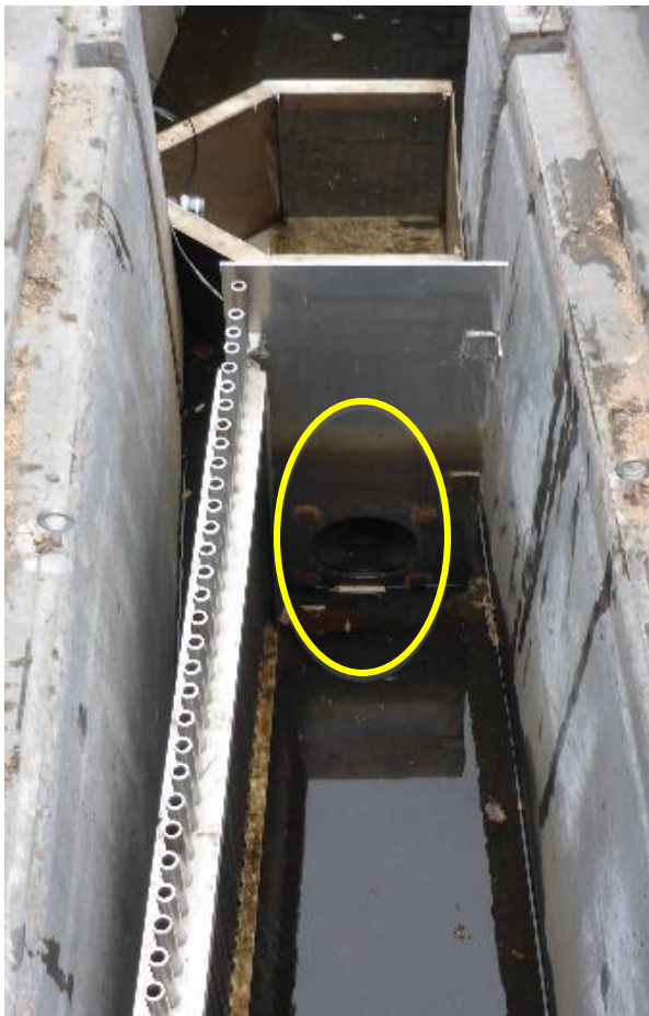
Photo 16: Entrance to the fish counter tunnel inside fish ladder (yellow circle)
