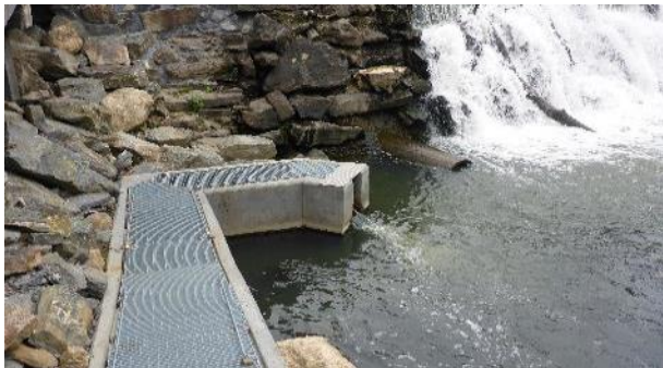
Photo 4: Fish entrance to the fish ladder
