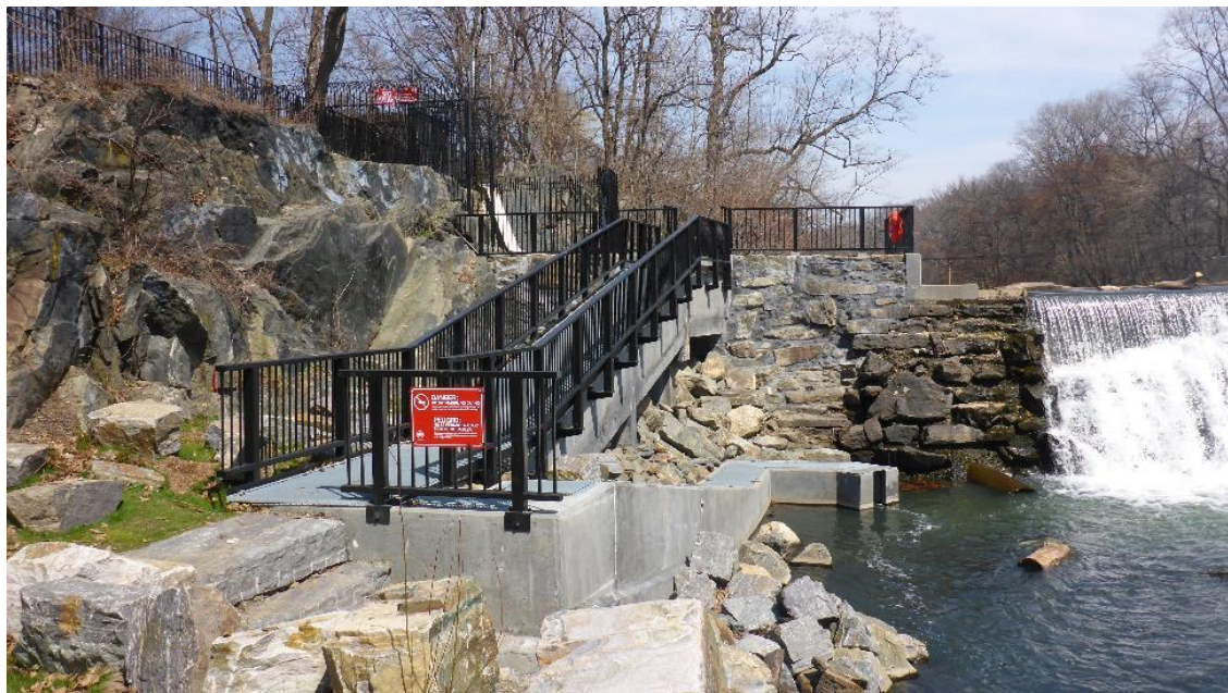
Photo 1: View of the river herring fish ladder at the East 182 nd Street Dam and adjacent to River Park
