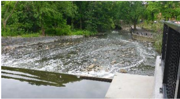
Photo 3: Looking downstream from top of the East 182 nd Street Dam
