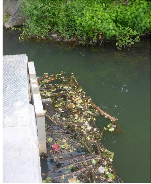
Photo 6: Fish exitway from fish ladder (side view)
