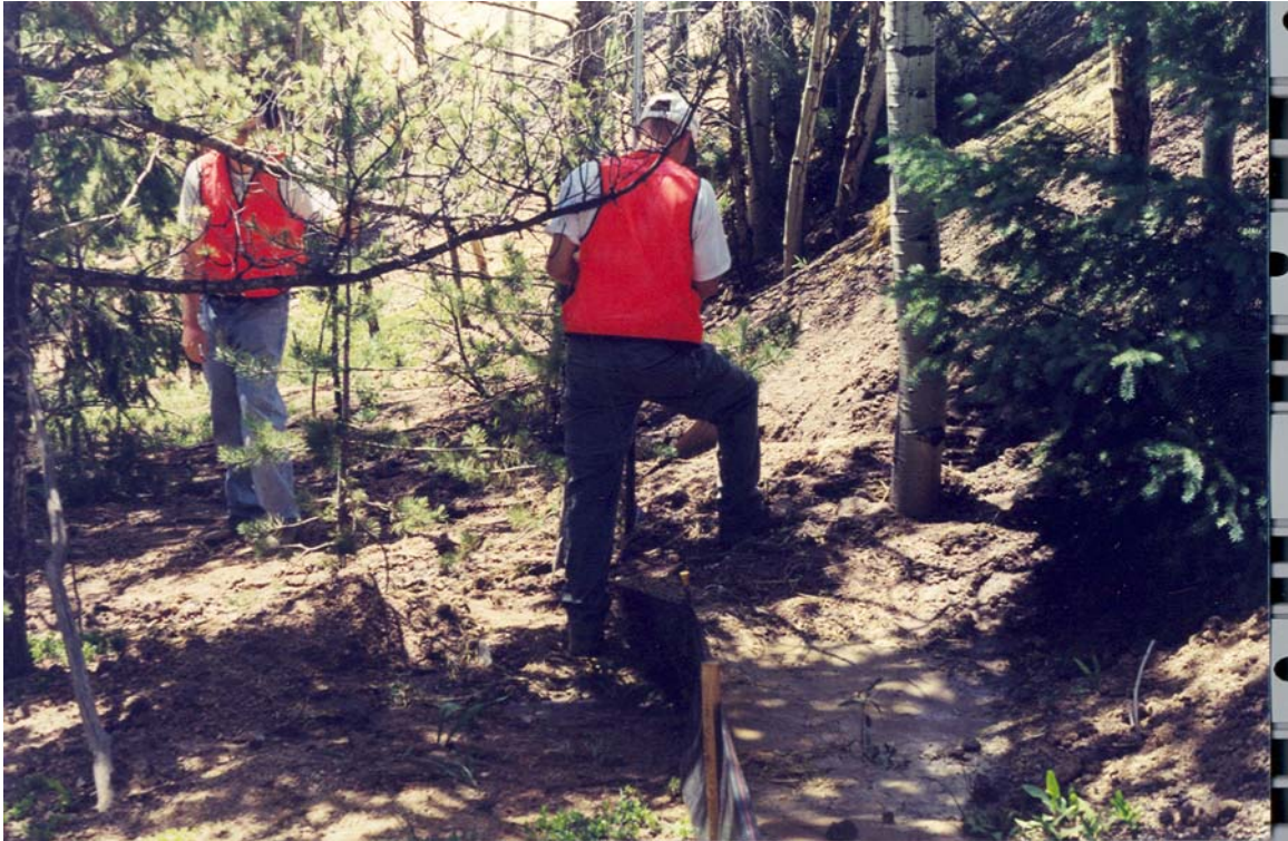
Figure 2. Surveying fill slope material in 007FS upper fence, June 30, 2003.
