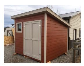
Built by the Capital Highschool carpentry class, this is not your everyday storage shed. It is 10' by 10' and built for all your needs with 5' doors to accommodate lawn mowers and 4-wheelers. High quality 2x4 construction @ 16" on center. Pre-finished Hardi plank siding, and architectural Land Mark, "Heather" shingles. It is fitted with a 2' by 2' window for natural light.
