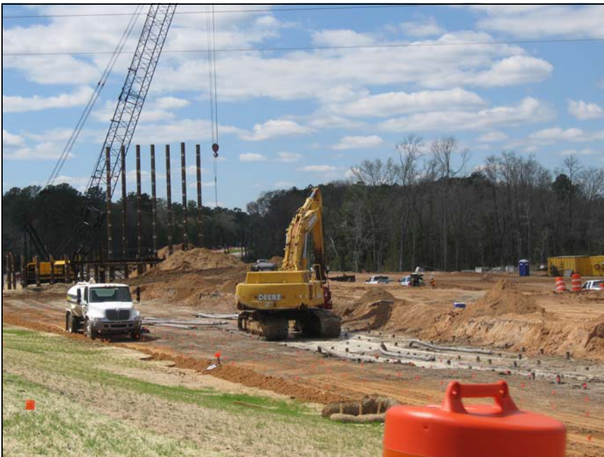
Construction at the US-17/US-21 Intersection
