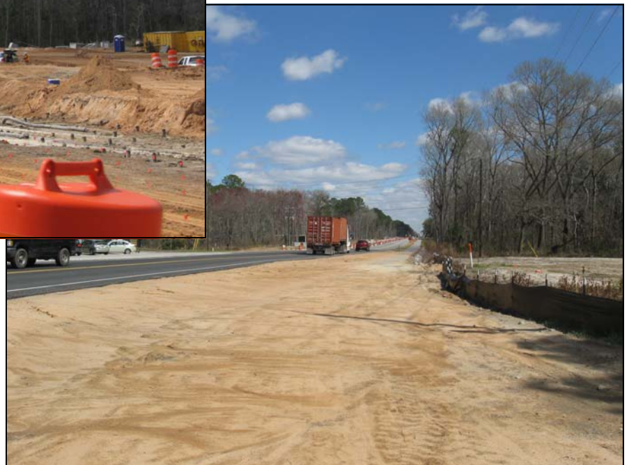
Embankment Build-up for Future Travel Lanes
