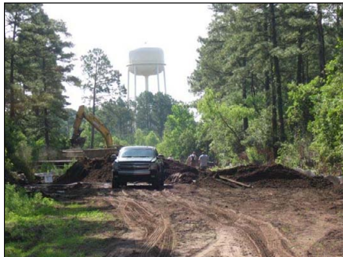
Water Line Relocation Along the Proposed Project Route
