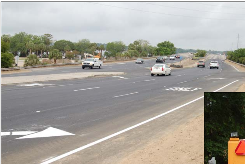
Completed Pinckney Island Portion of the Project
