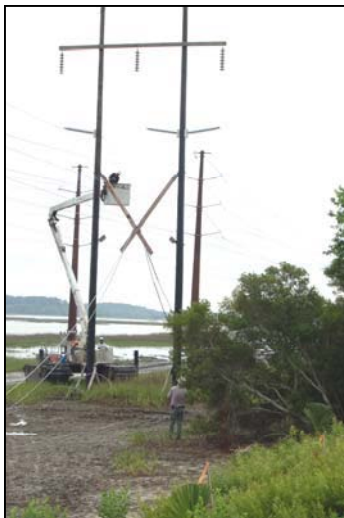
Santee Cooper Removing Abandoned Power Poles
