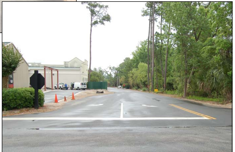
Completed Paving for New Frontage Road
