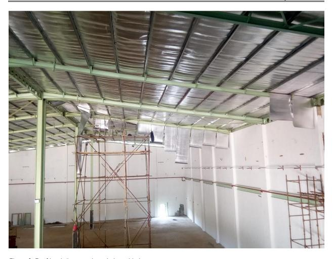
Figure 3. Roof insulation- new layer being added
