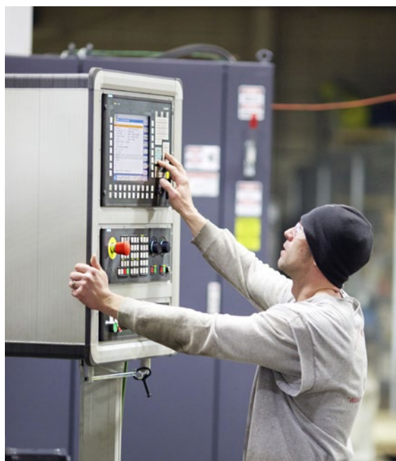
Three Sinumerik CNCs, plus a PLC, run the entire system
