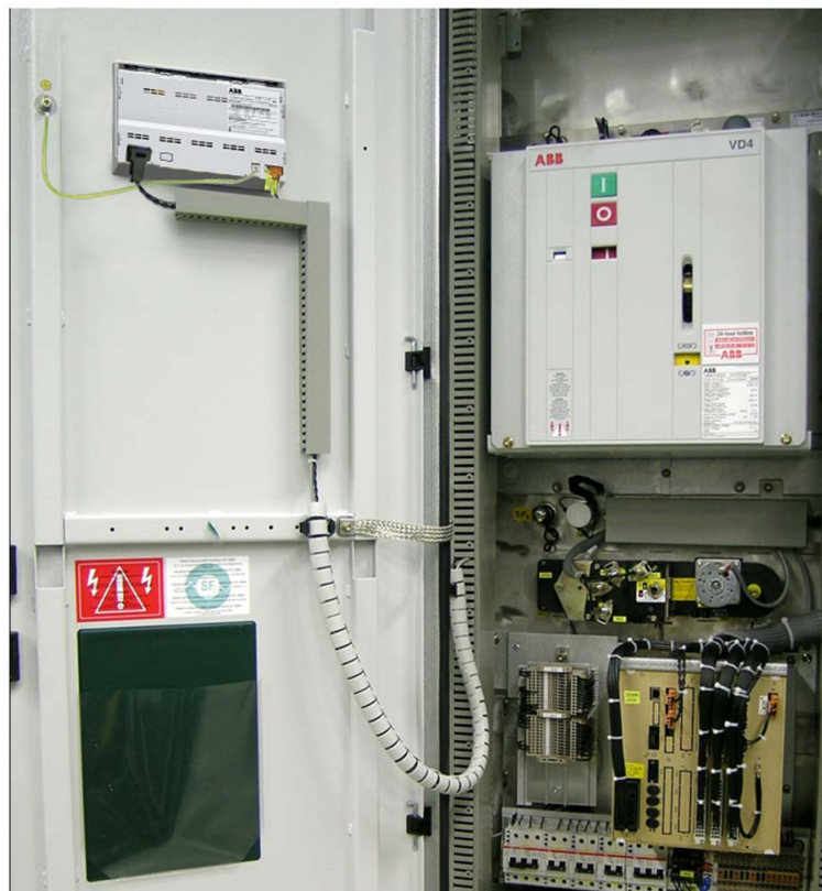
Fig. 6.2.2.-3 Example of mounting of the Central Unit in the LV compartment and the HMI on the door
