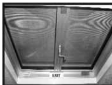
Emergency Exit Ceiling Vent
