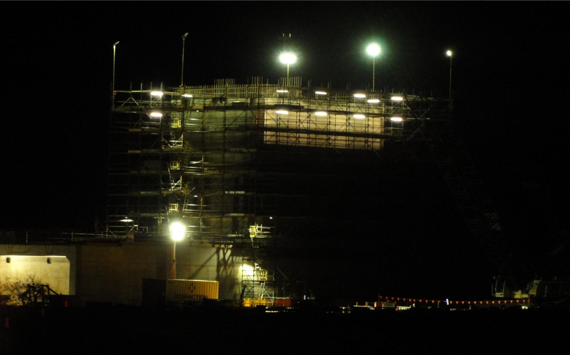
BOO primary crusher under construction
