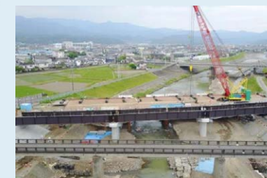
Repair work on the Kyudai Main Line
