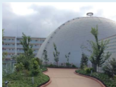
Greened sections of Ropponmatsu 421's roof
