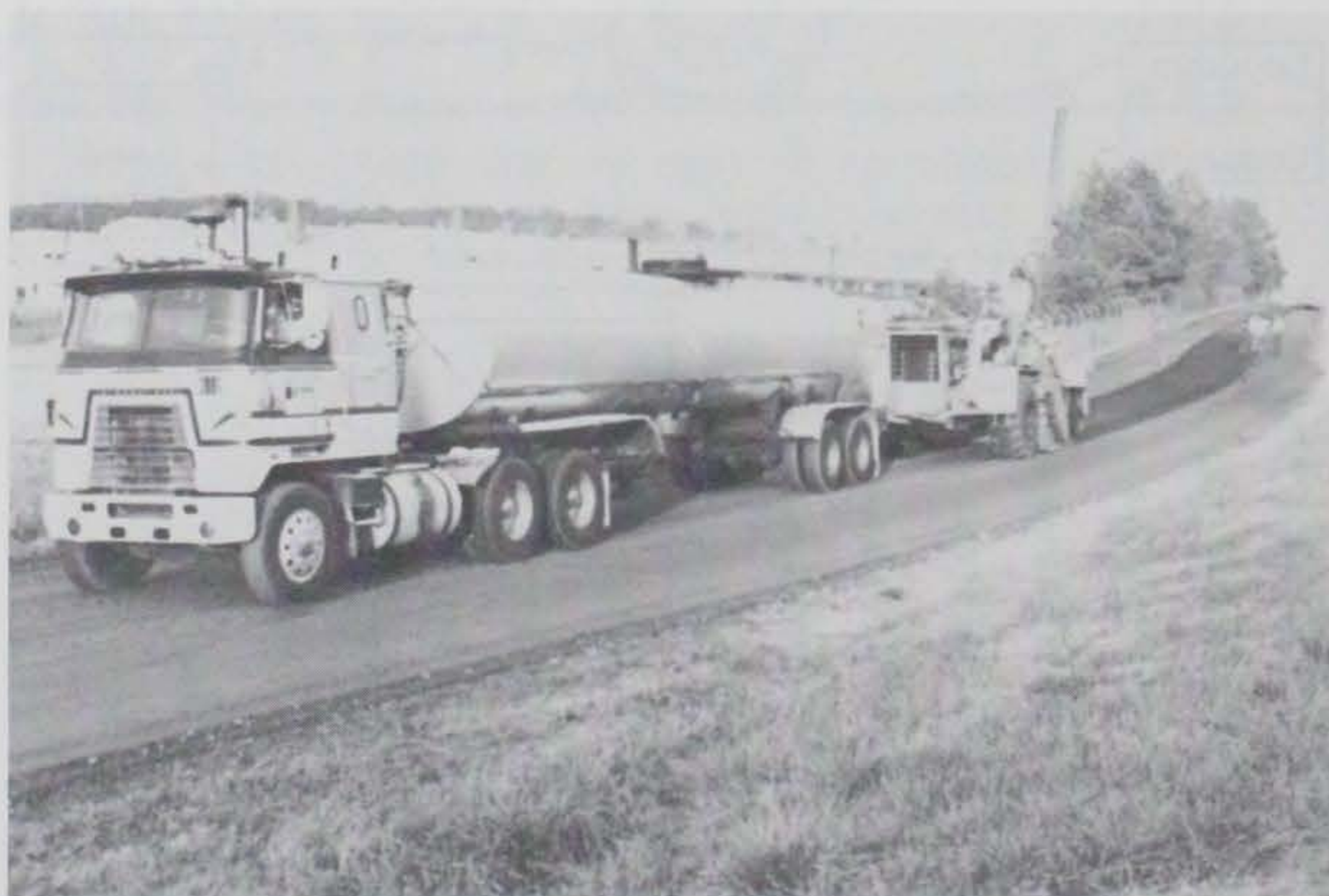
Figure 14. Mixed-in-place cold-mix recycling
