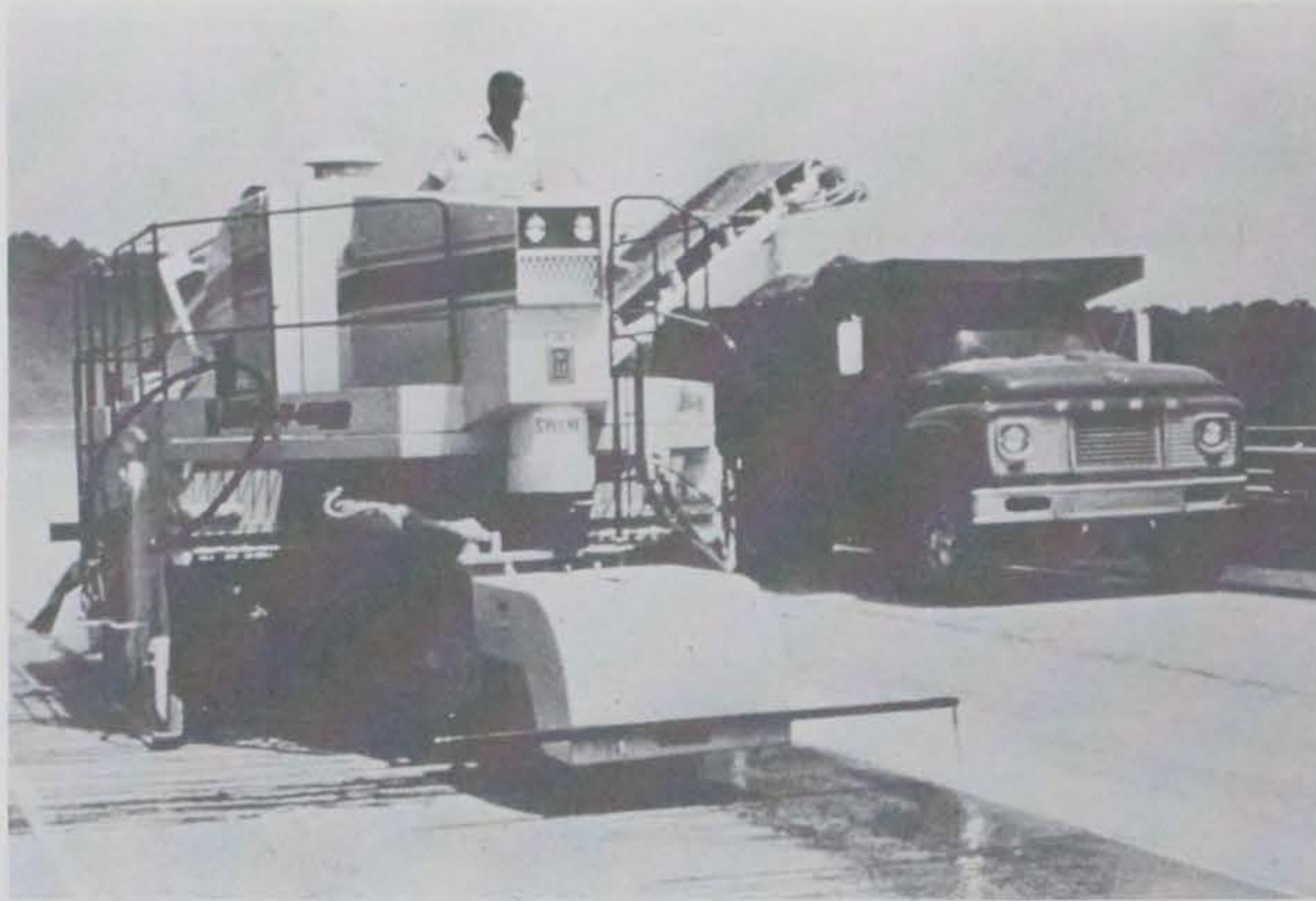
Figure 7. Example of equipment (cold-milling machine) used to remove pavement to desired depth, grade, and/or slope
