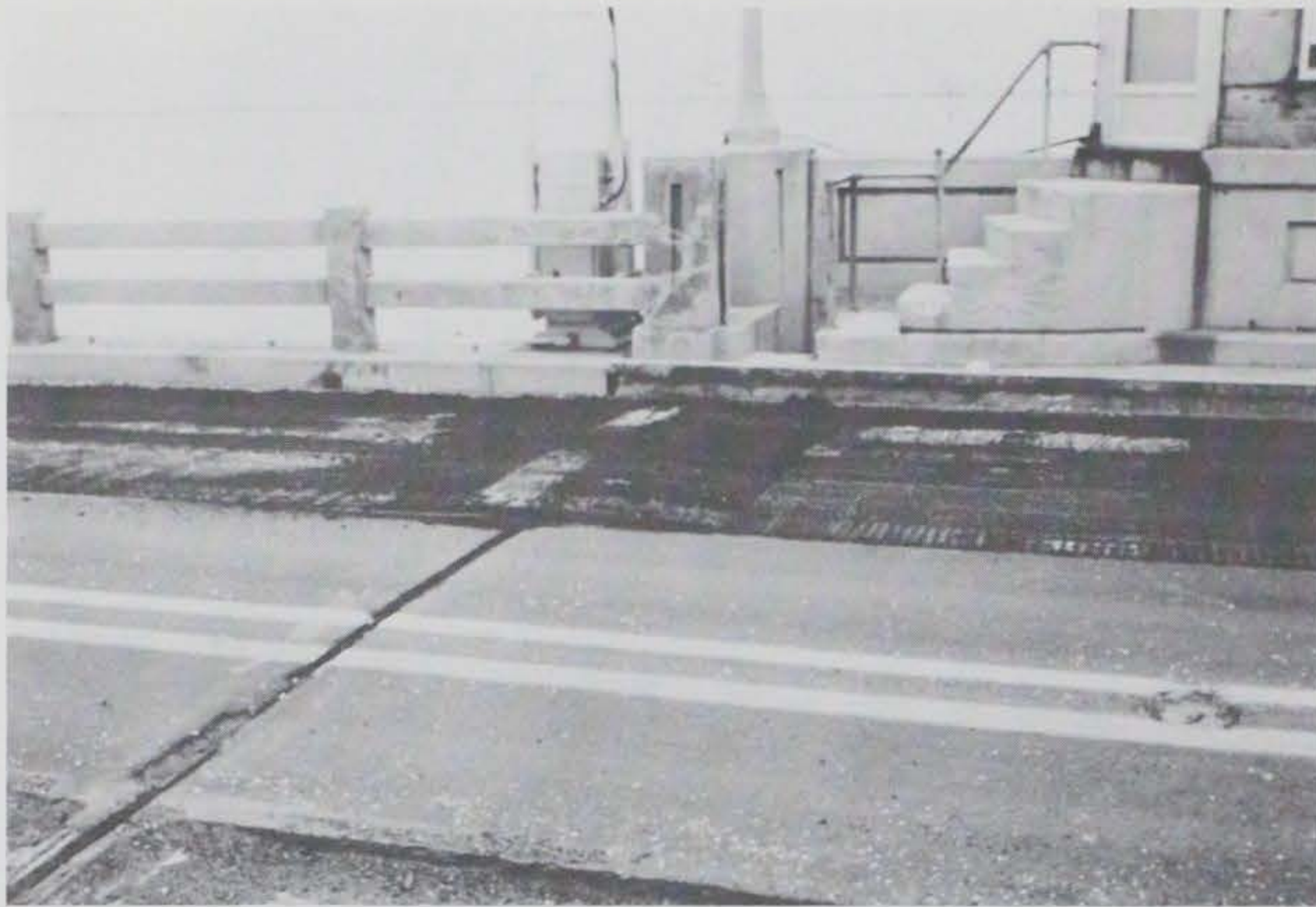
Figure 22. Removing pavement from bridge to maintain allowable dead load
