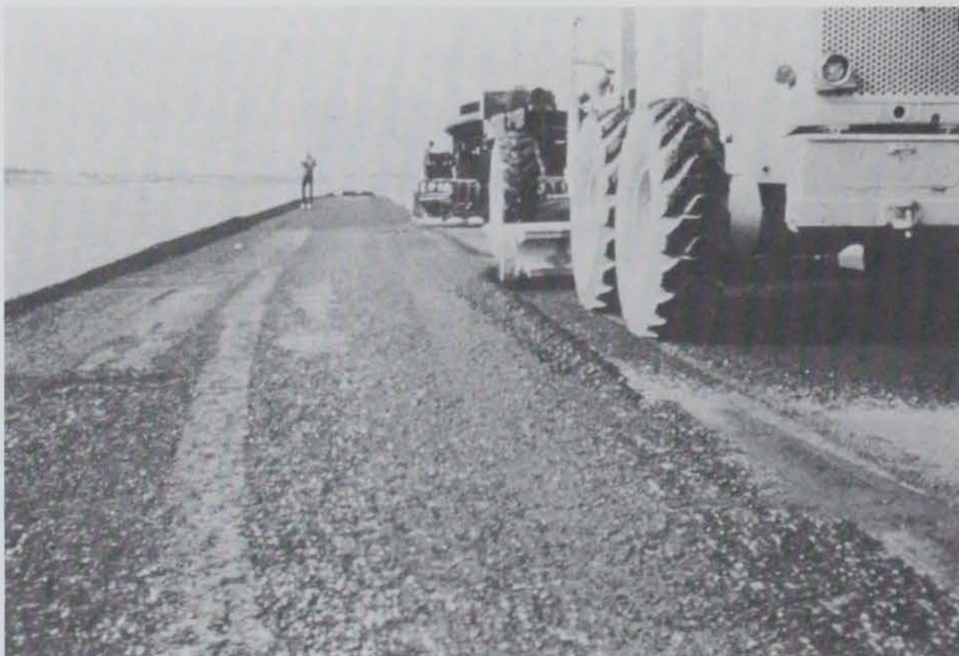
Figure 4. Planer operation following a heater-scarifier
