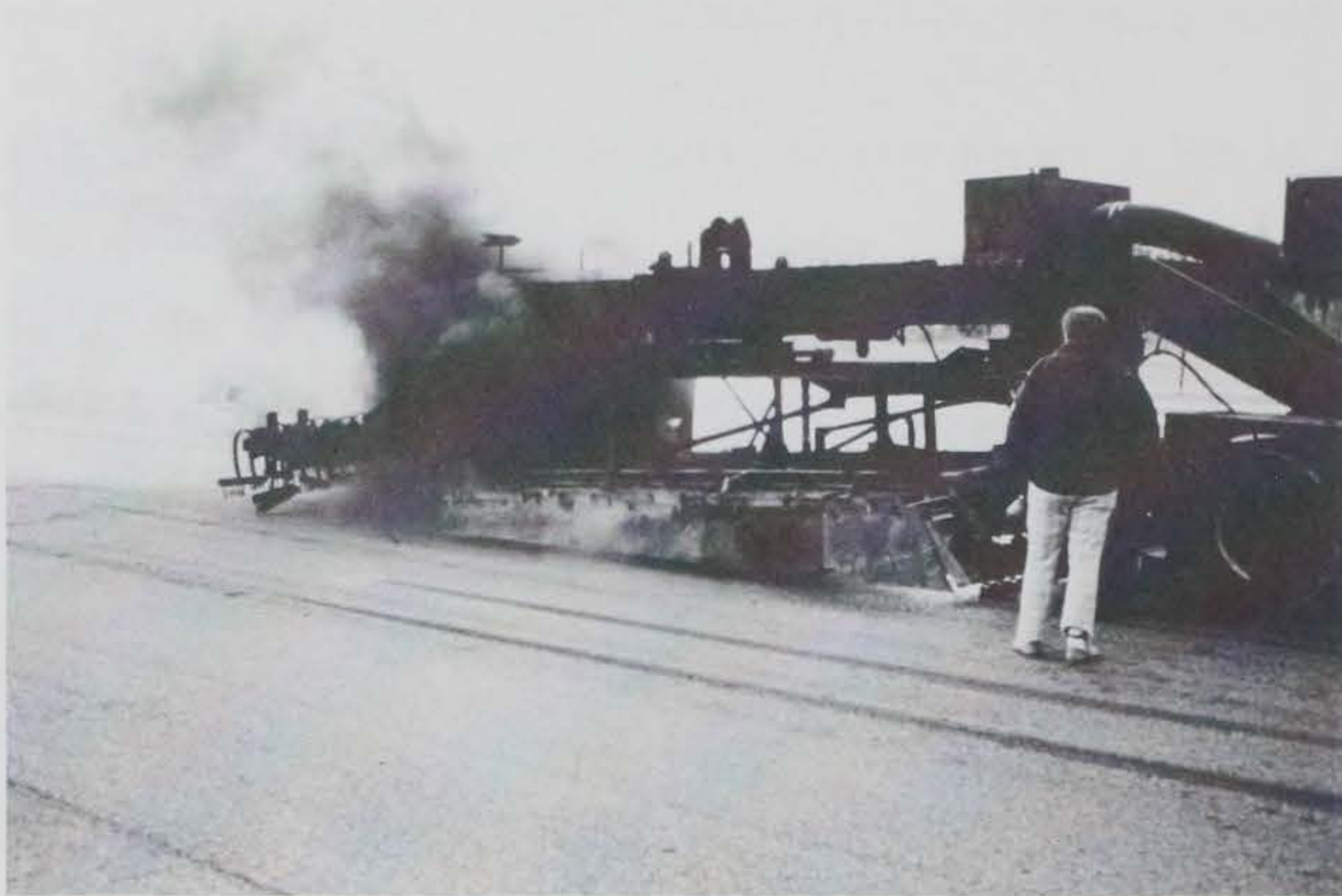
Figure 3. Heating and scarifying operation
