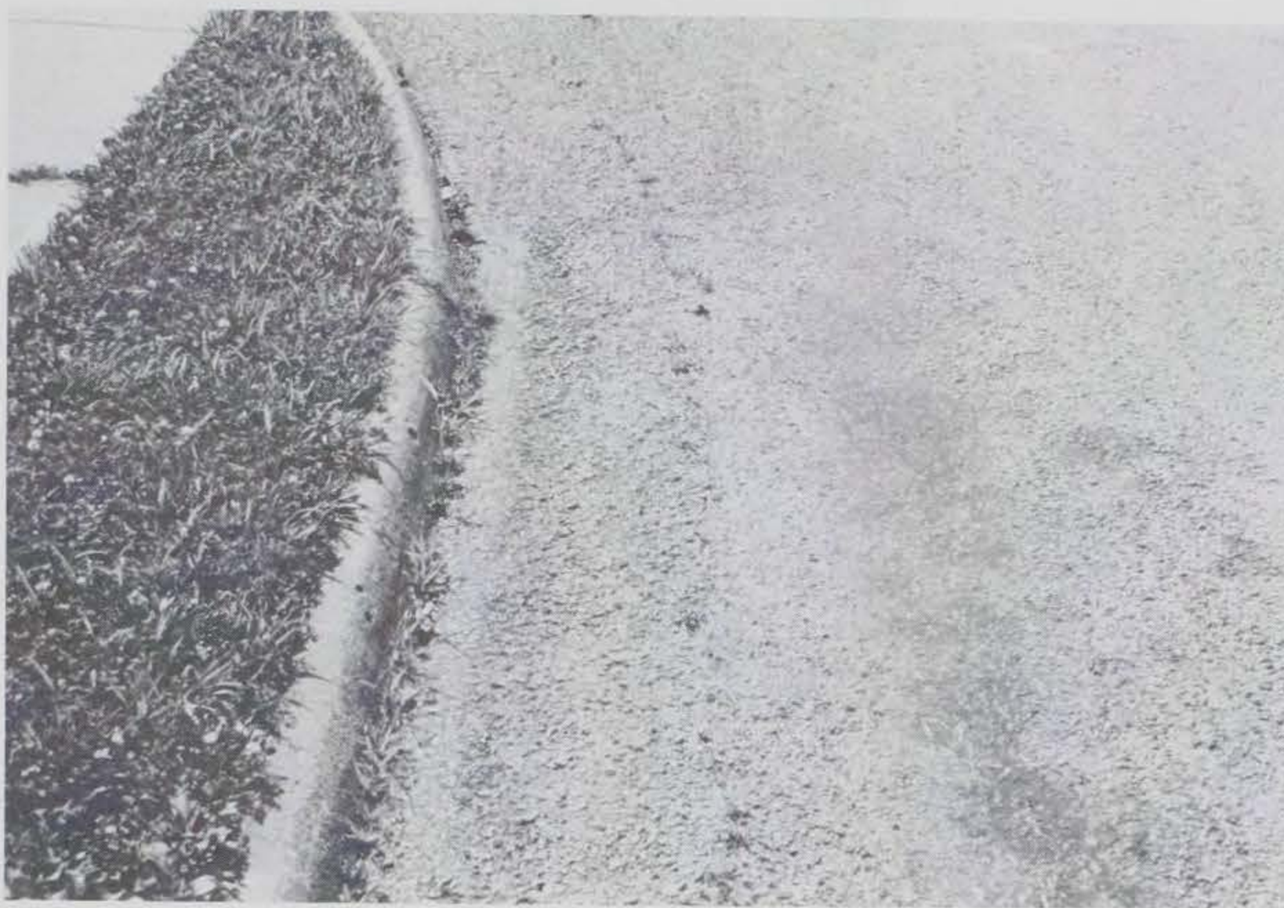
Figure 24. Asphalt overlay placed over concrete curb and gutter
