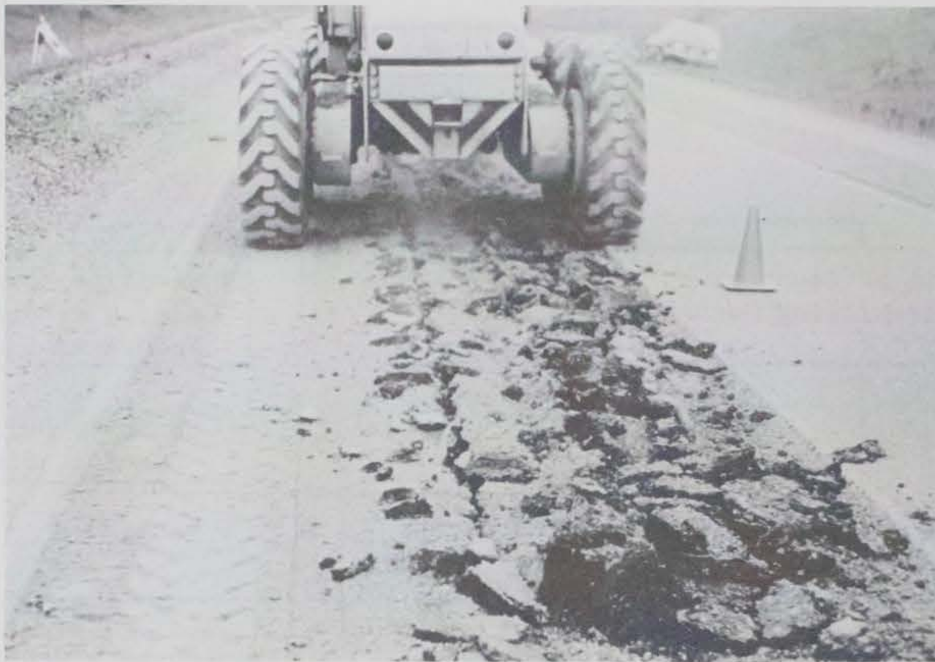
Figure 13. Ripping up pavement in preparation for cold-mix recycling
