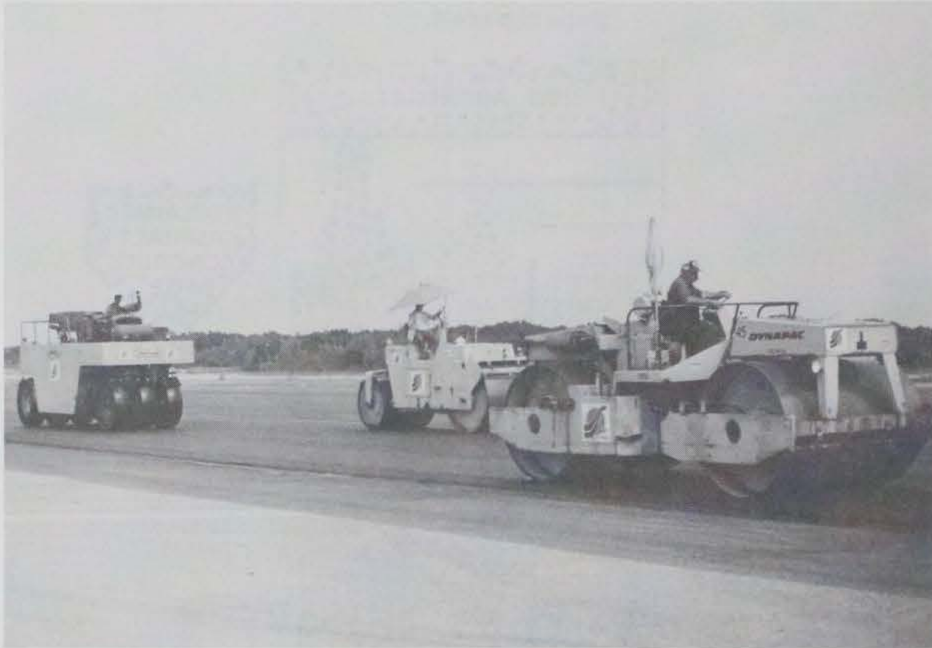
Figure 18. Rollers compacting a hot recycled pavement
