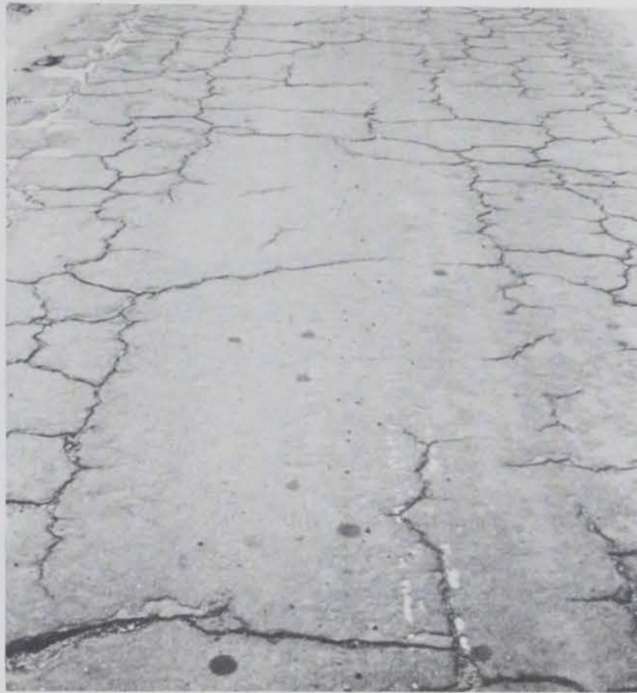
Figure 20. Abandoned road is an eyesore
