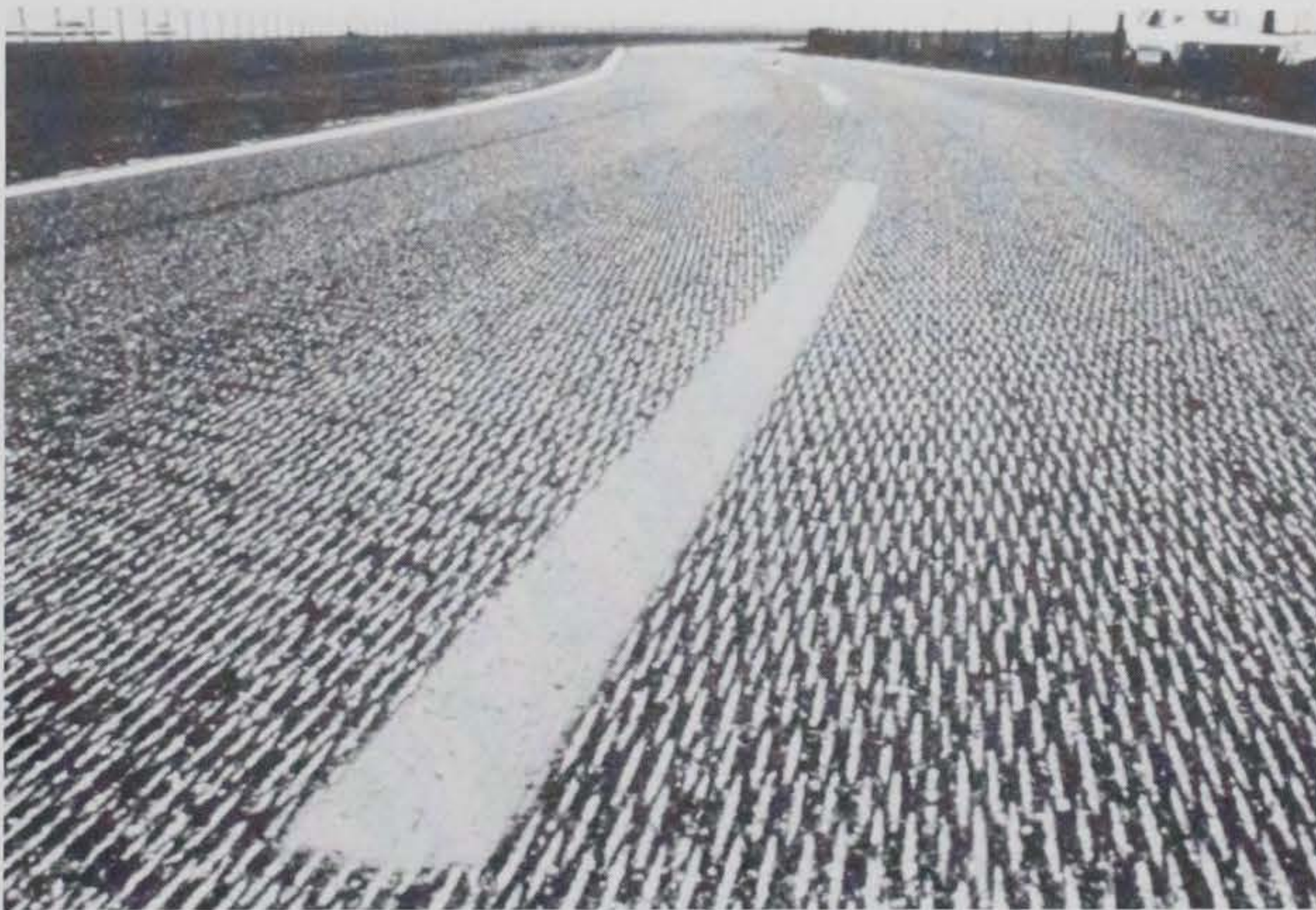
Figure 6. Surface texture produced by cold milling
