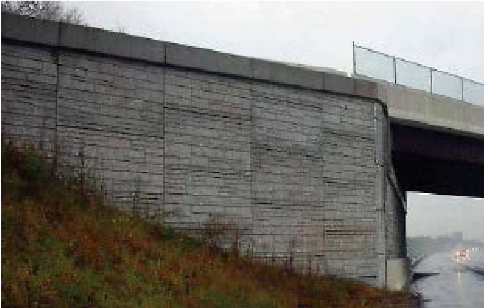
Indiana Toll Road Improvement in Gary
