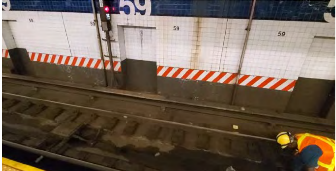
Figure L-4. ST Signal at 59th Street-Columbus Circle Station.
