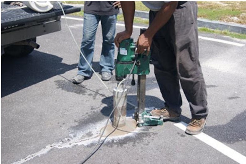
Figure 27. Drilling of paved surface for coring test
