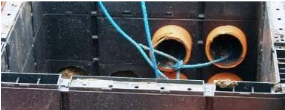
Figure 22. Draw rope inside duct
