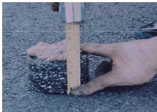
Figure 28. Measuring of asphalt premix thickness
