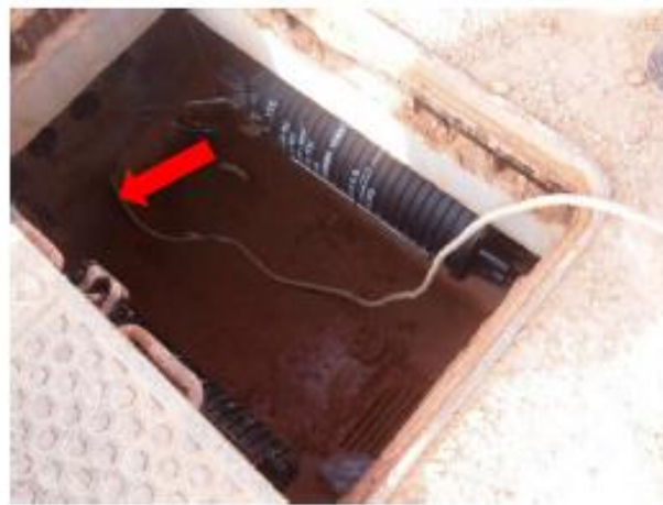
Figure 25. Mandrel test point at terminated manhole
