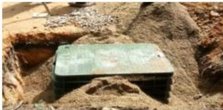
Figure 14. Manhole backfilling
