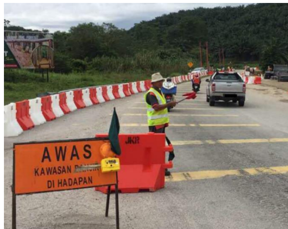
Figure 2. Flagman to control traffic
