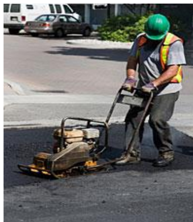
Figure 29. Compacting of asphalt premix
