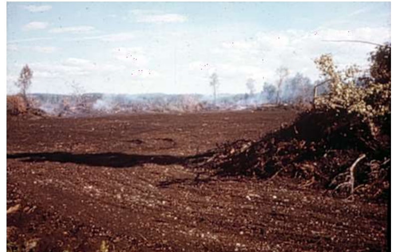
Clearing muck soil in Cookstown Marsh
