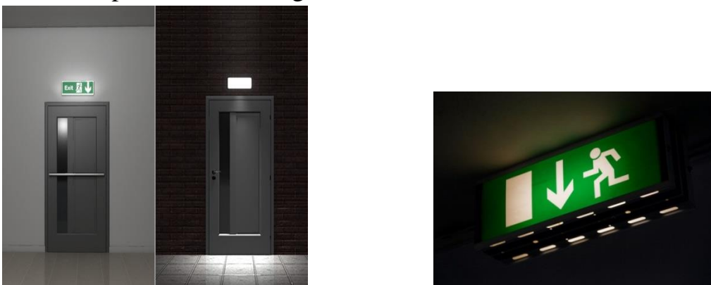
Figure 6-1: Emergency lighting in building to final exit.
