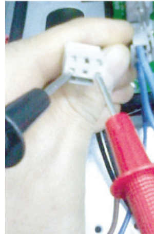
< Checking the Press switch >
