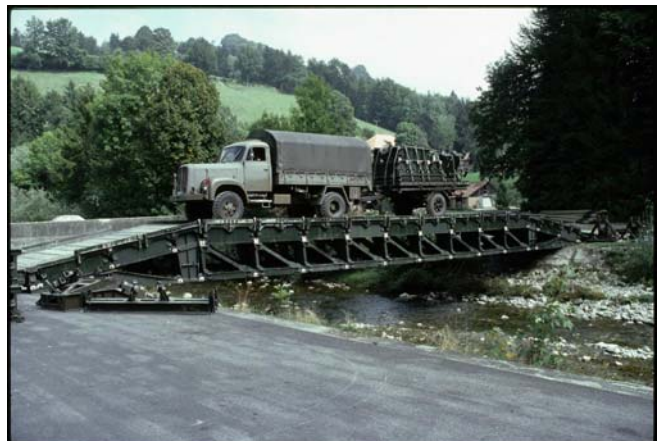
Figure 3: The Medium Girder Bridge being used by the Swiss Army. From Swiss Military website, http://zem.dev.imagefinder.ch .
