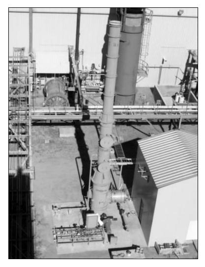
Figure 3. Photograph of NO<sub>x</sub>idizer<sup>™</sup> installed at MSE Technology Applications in Butte, MT.
