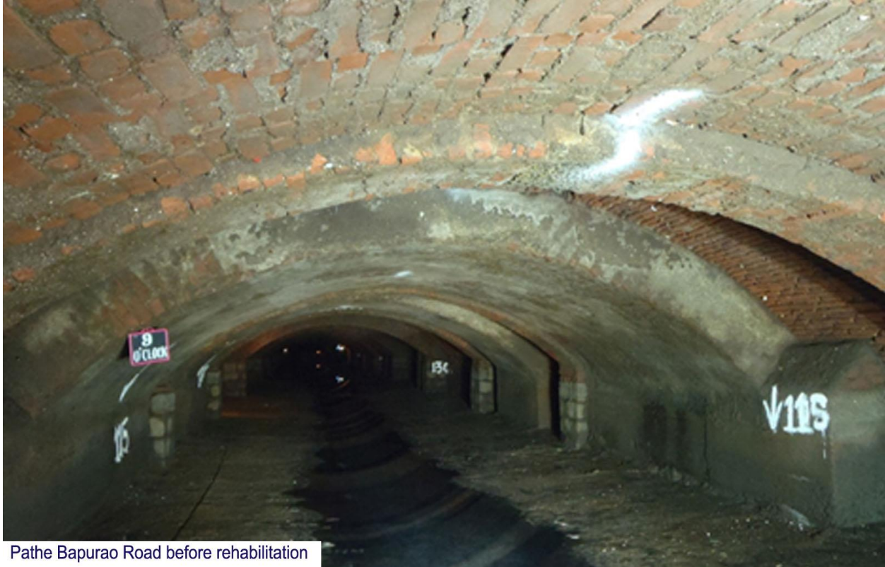
Figure 5: Rehabilitation of underground storm water drains
