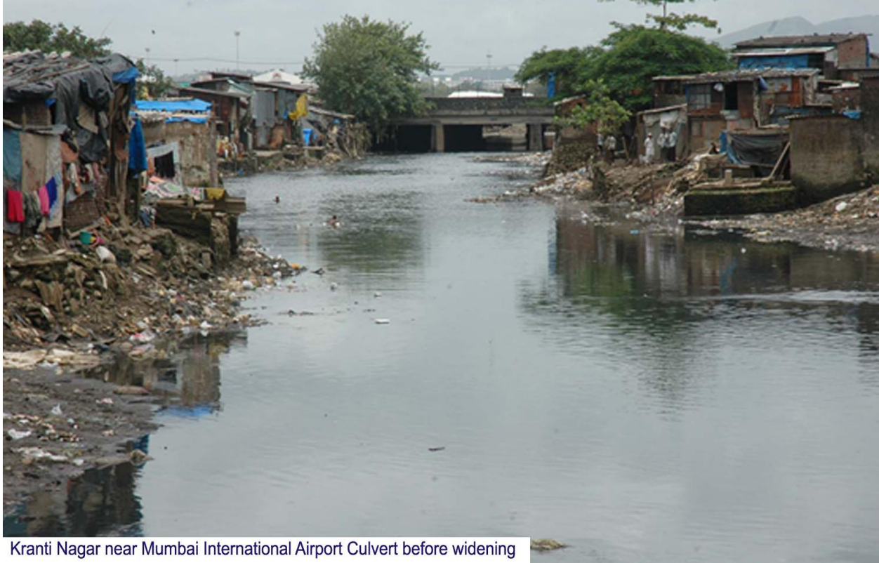
Figure 7: Widening of open storm water drains
