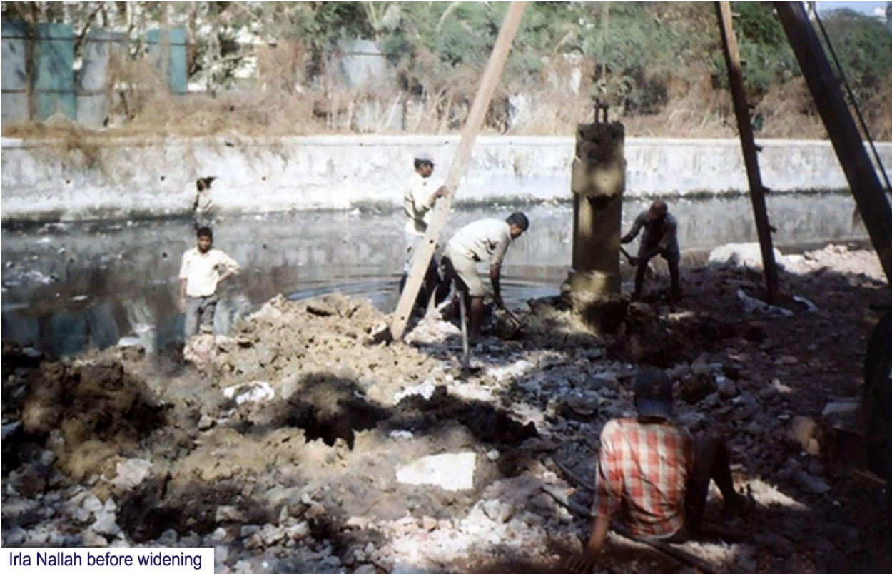
Figure 2: Widening of storm water drains
