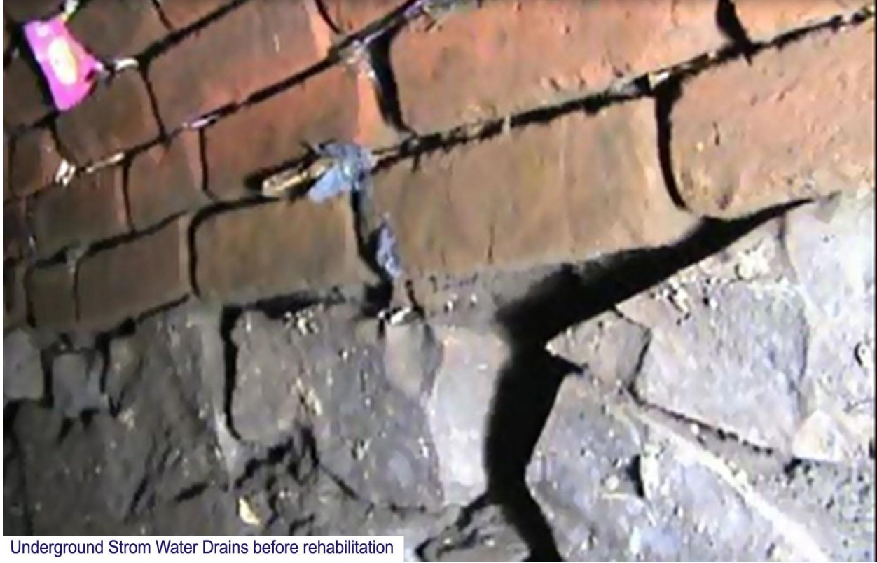
Figure 6: Rehabilitation of underground storm water drains
