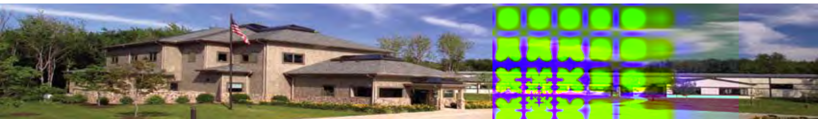
Snap-tite's Corporate Office and one of six manufacturing facilities centrally located near Erie, Pennsylvania, USA.
