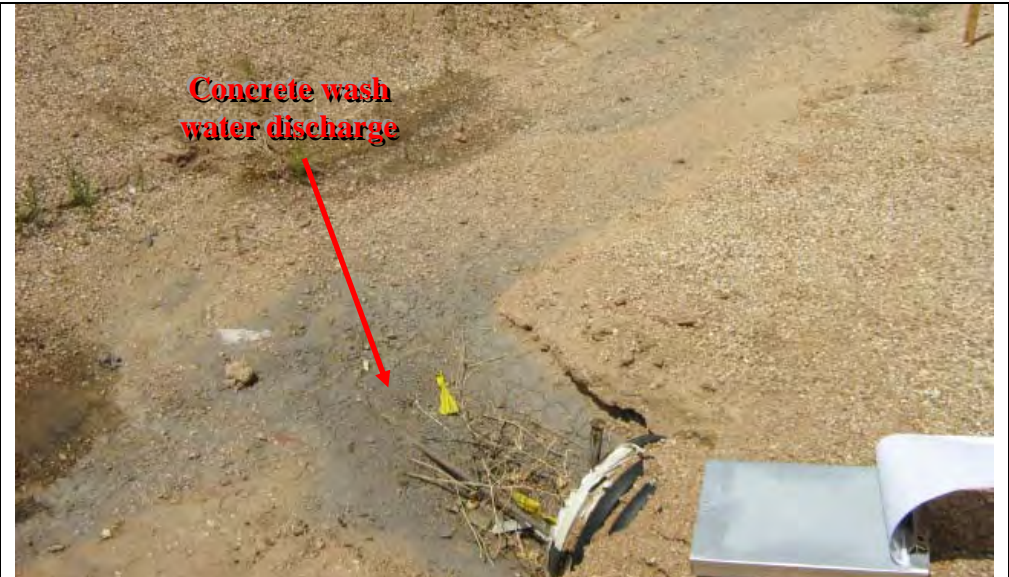
Photograph 2 – Close-up view of outlet shown in Photograph 1
