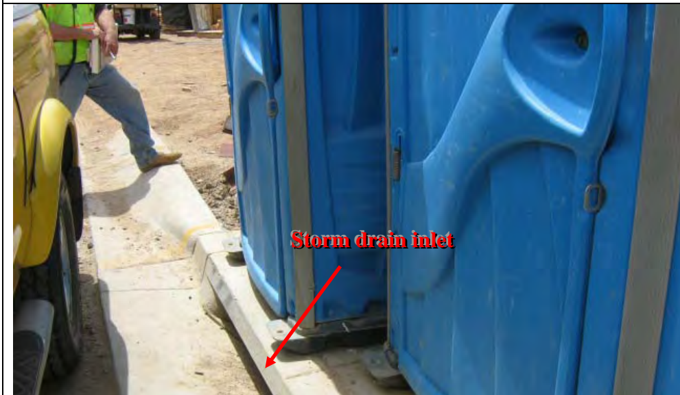
Photograph 11 – Portable toilet improperly placed directly adjacent to inlet
