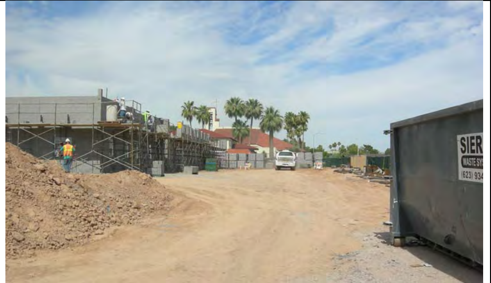
Photograph 2 – View from construction site entrance to the west.
