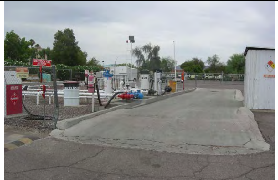
Photograph 2— View of truck fueling station
