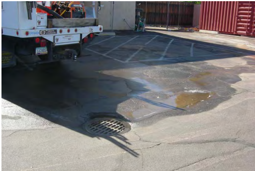
Photograph 10. Wash water entering storm drain from a water department vehicle.
