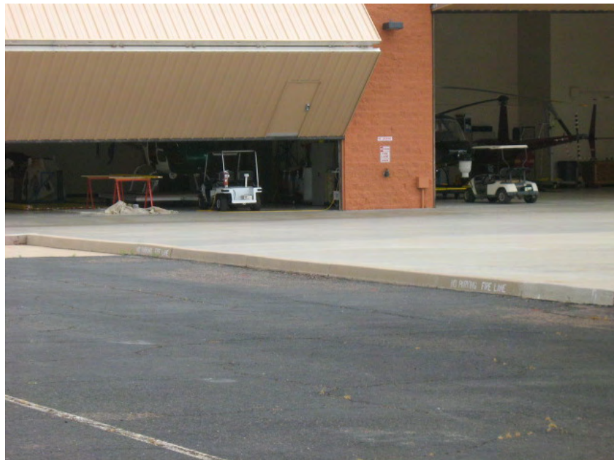
Photograph 2. Scottsdale Airpark – Industrial activities such as aircraft service and storage were observed at the Westcor Aviation facility.
