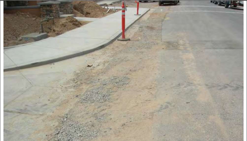
Photograph 2 – View facing south on Woodmere Fairway adjacent to Phase I site entrance.
