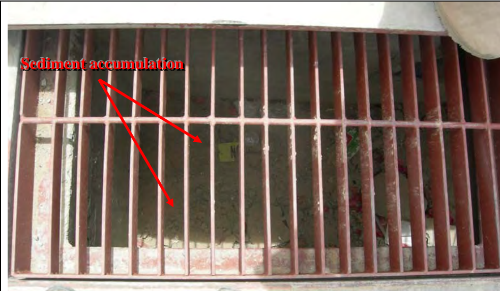
Photograph 1 – View of storm drain inlet along Woodmere Fairway.
