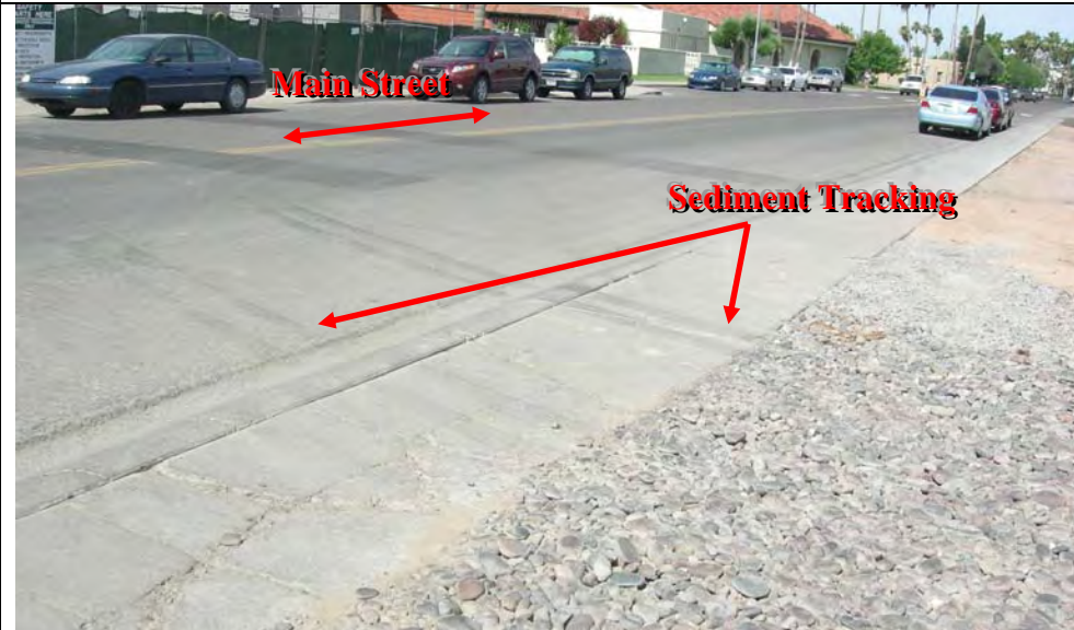
Photograph 3 – View of vehicle tracking onto Main Street, facing northeast.
