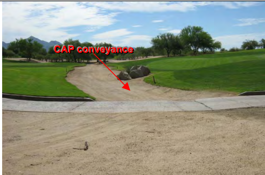
Photograph 1 - Central Arizona Project (CAP) conveyance
