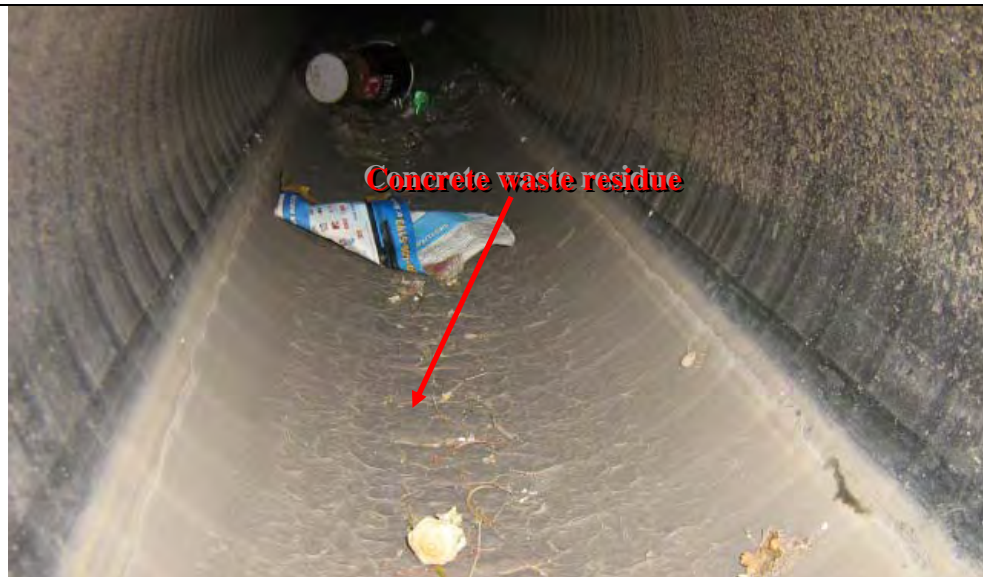
Photograph 3 – View inside outlet pipe shown in previous photographs
