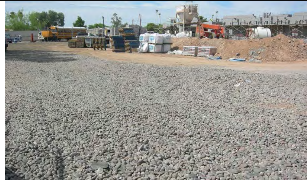
Photograph 1 – View of construction entrance facing south.
