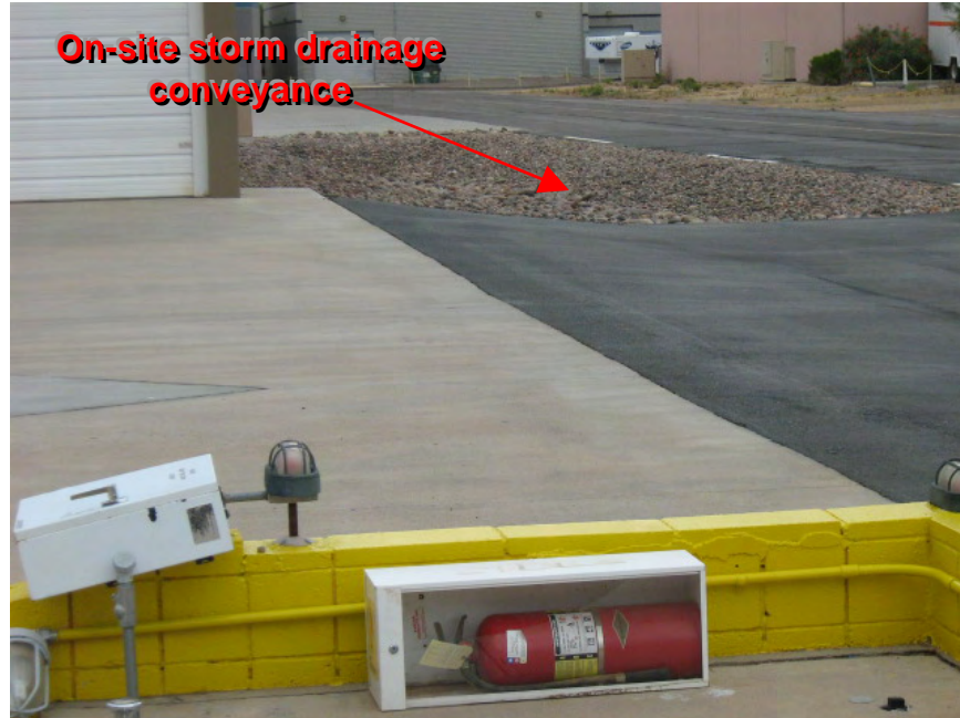
Photograph 5. Scottsdale Airpark – View of Aircraft fueling system located northeast of 7916 East Beck Lane; potential for spills and subsequent conveyance to storm drain system.
