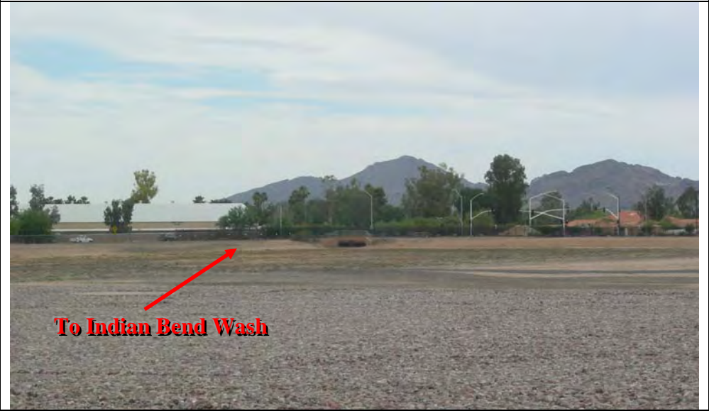
Photograph 4—View of airport detention basin, facing southeast
