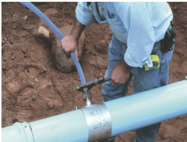
Fig. 11: Angle MUNICIPEX pipe 10 to 20° above horizontal at connection to water main
